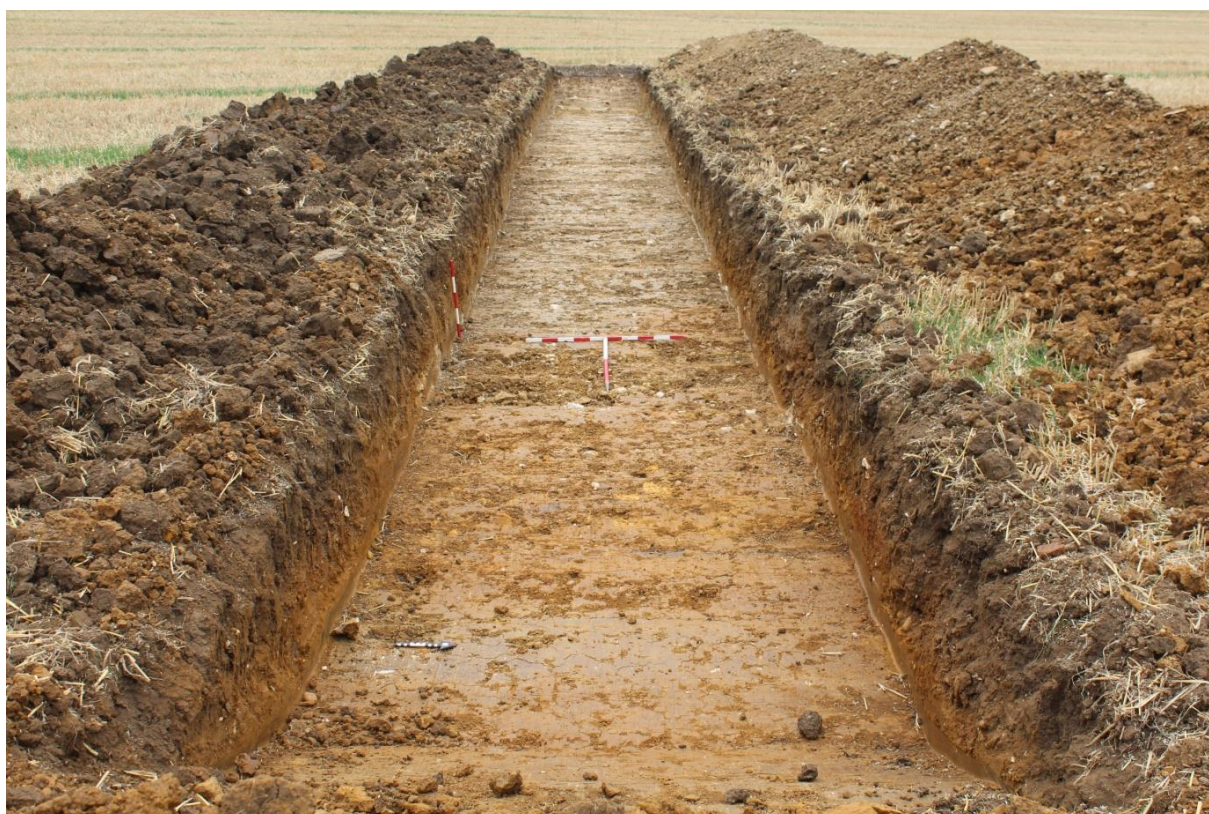
Plate 2: View of trench 7 looking west, demonstrating the variation in the natural deposits on the site.
