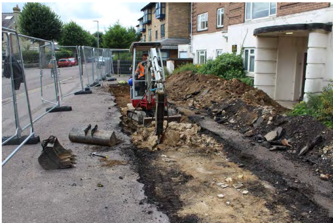
Plate 2: Trench 1, machining, view west
