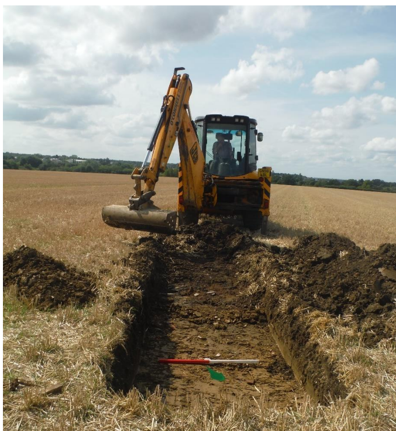
Plate 2 Trench 6; view west.
