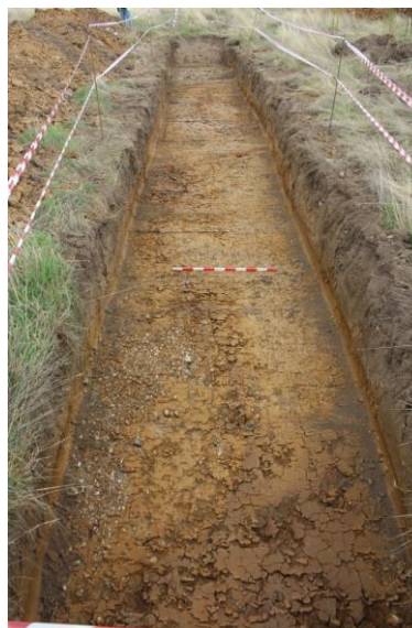
Plate 3: Trench 3 – Looking South-East
