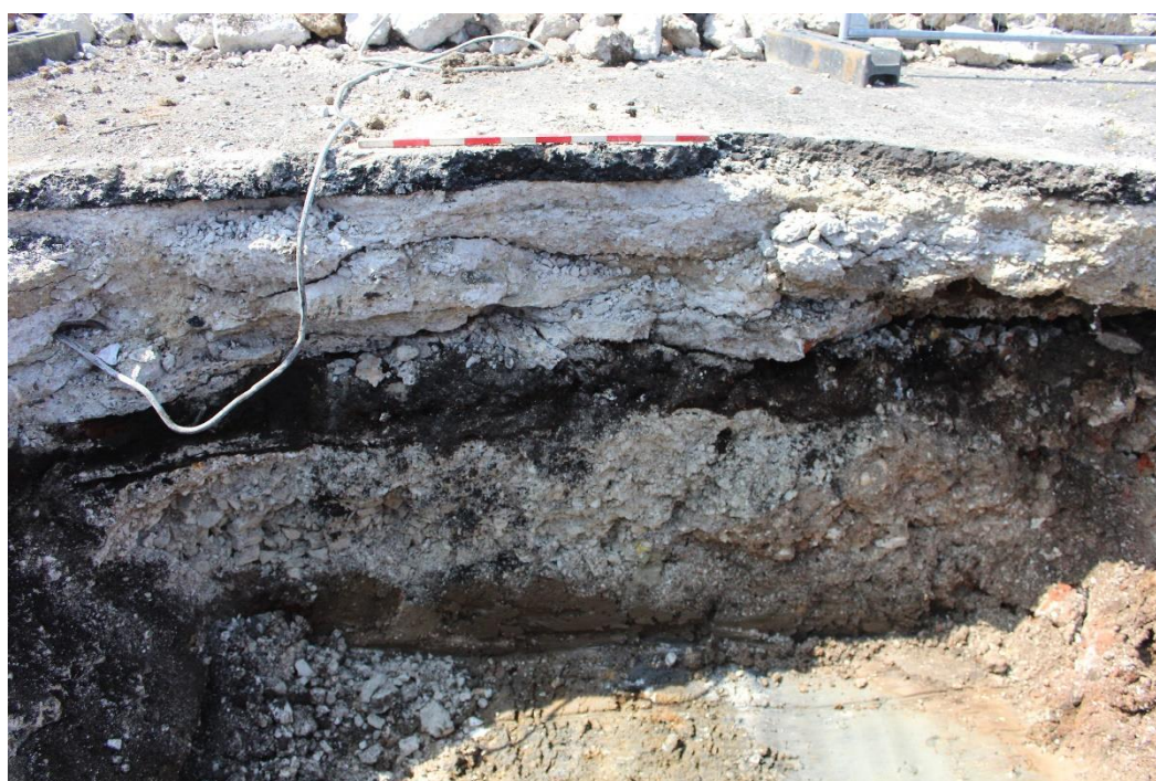
Plate 1: North-east facing section 1 in Trench 2 (1m scale)
