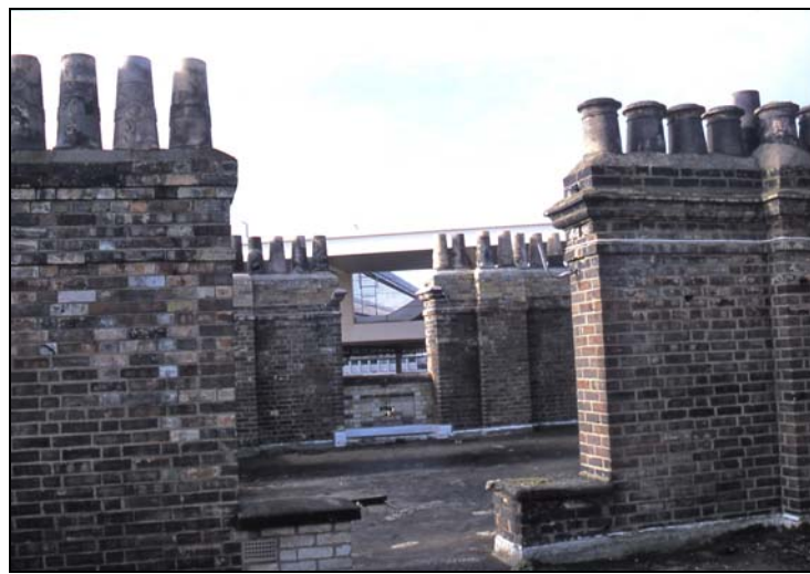
Plate 8: View of the roof, looking south-west
