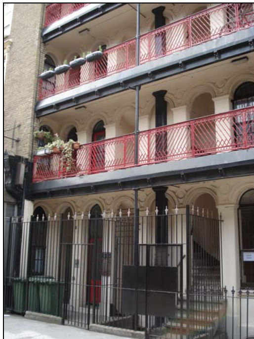
Plate 23: The Cromwell Buildings, New Southwark Street: balcony detailing
