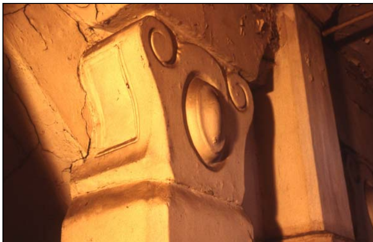
Plate 5: Detail of scroll-moulded impost on balcony
