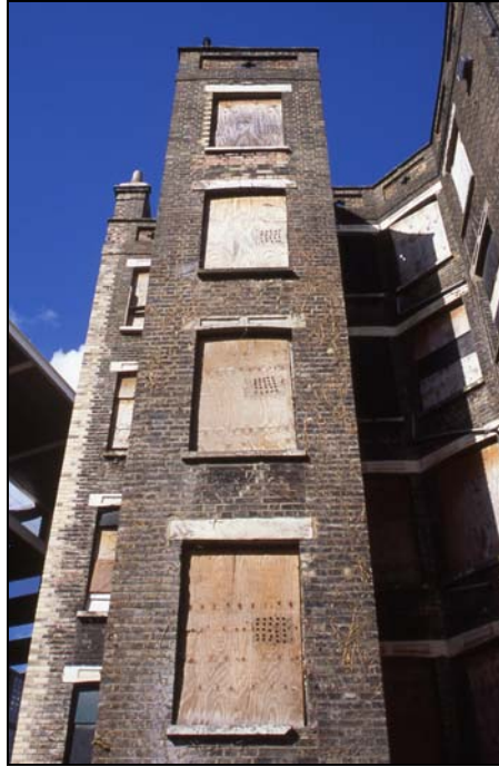
Plate 7: Southernmost rear extension, from the south-east
