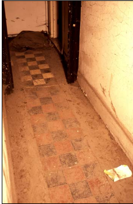
Plate 10: Original red, white and black tiles inset in access corridor concrete floor
