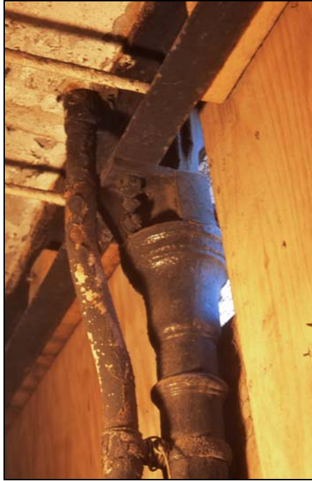
Plate 4: Detail of column-beam junction on balcony
