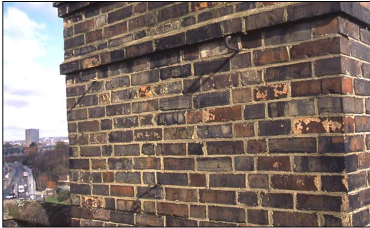
Plate 9: Clothes-line hooks on chimneystack
