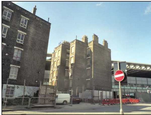
Plate 1: View of northern Stanley building from the east
