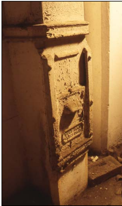
Plate 6: Detail of dust and ashes chute on balcony
