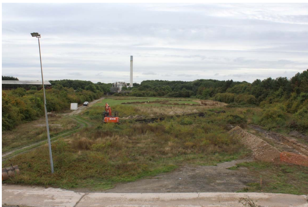
Plate 1: Area A, view east.
