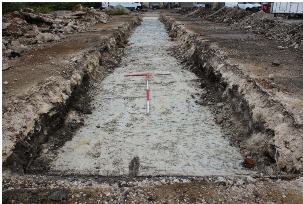
Plate 12: Trench 9, truncated natural chalk, view west.
