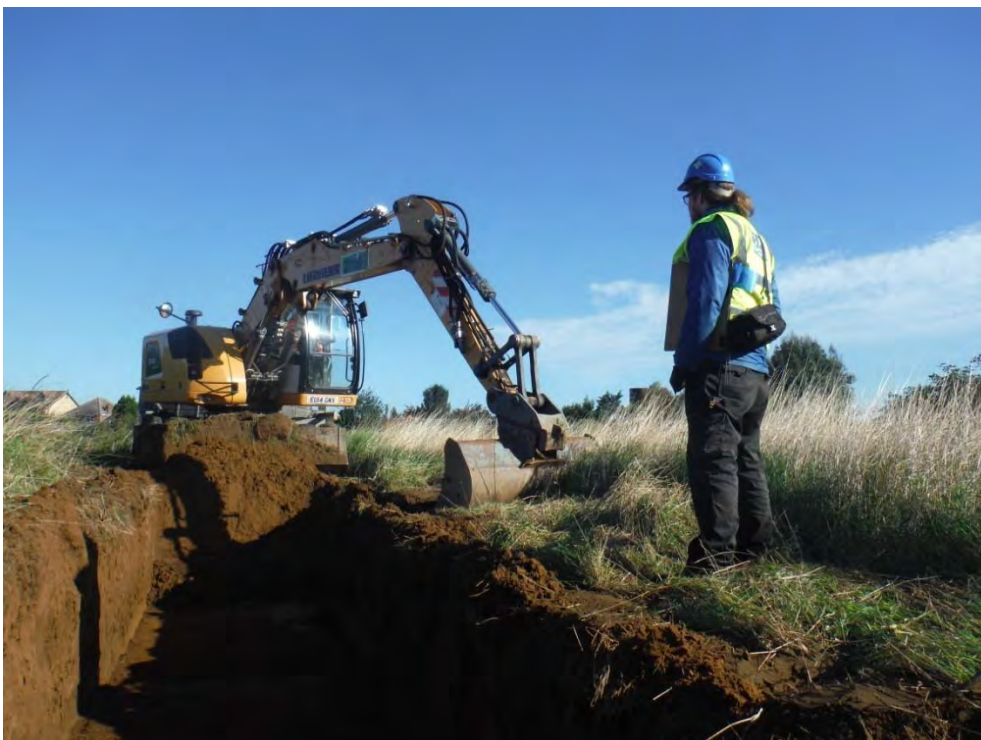
Plate 2: Machine excavation with a 360° tracked excavator
