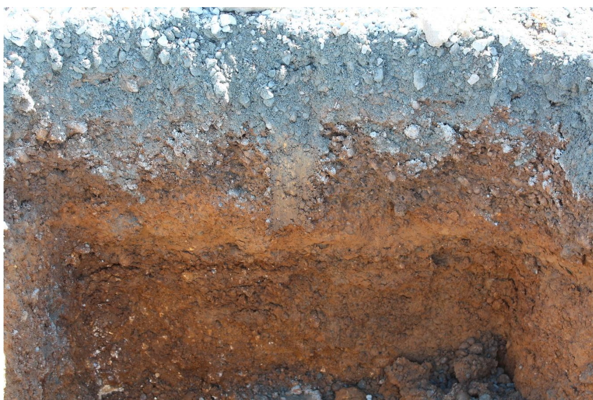
Plate 4: SE facing section of Trench 36
