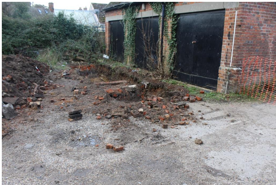
Plate 3: Trench 1 and existing garage building
