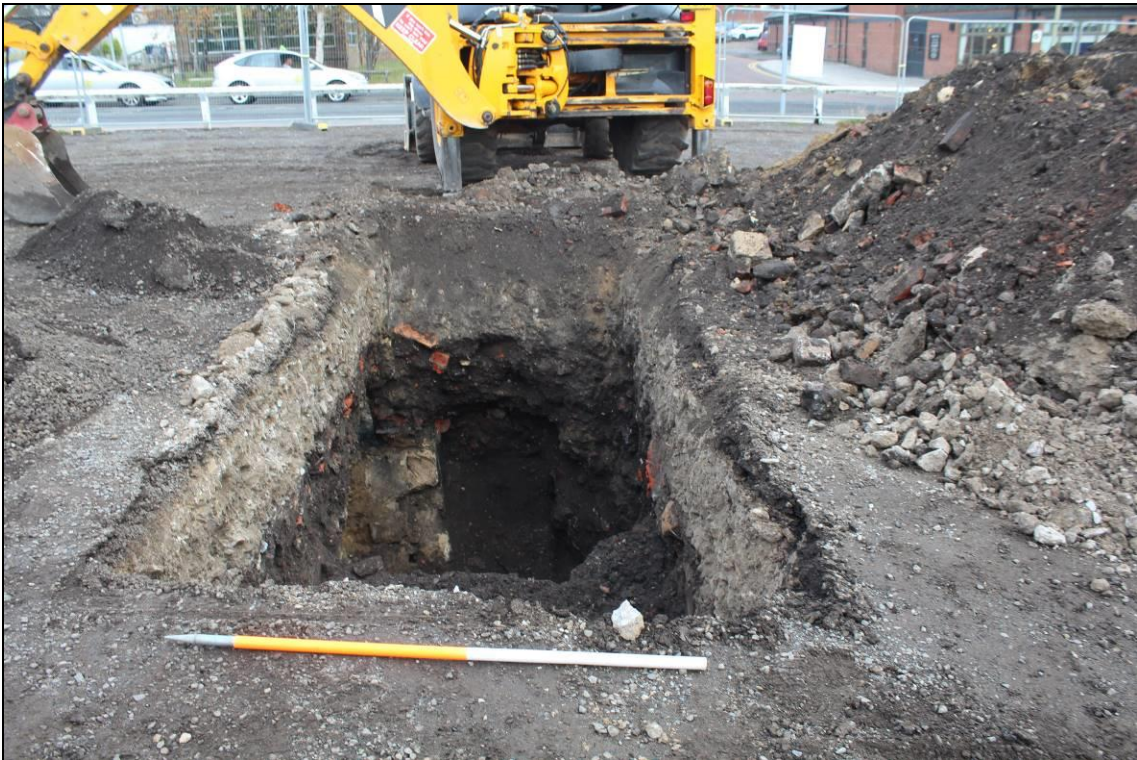
Plate 3: Trench 3, wall [304] in east section: view east, scale: 1m
