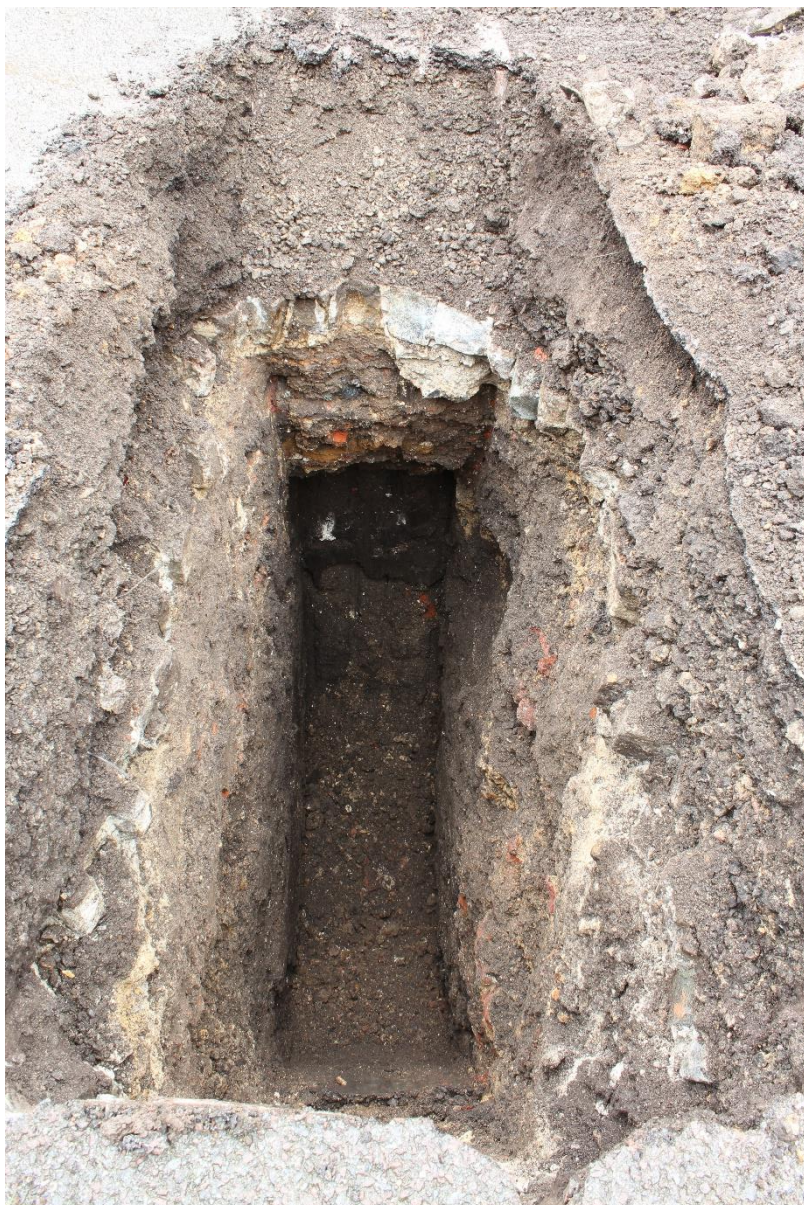
Plate 1: west facing photograph of Trial Pit 2
