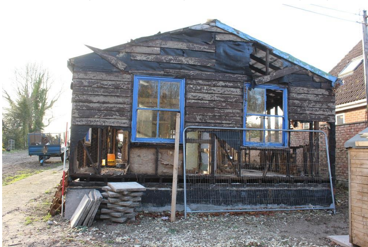
Plate 6: North-north-west facing view of north-east facing frontage. 2m scale
