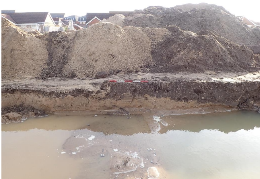
Plate 1: View to east Trench 1, 1m scale
