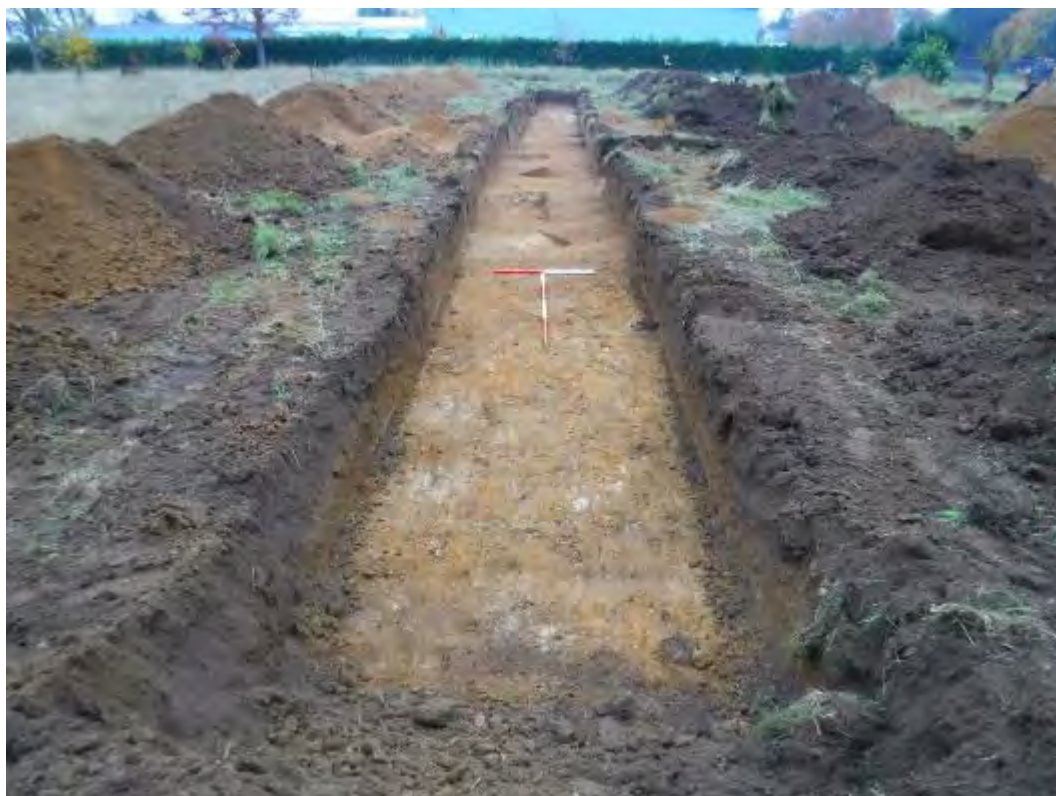
Plate 5: Trench 5, view south-east
