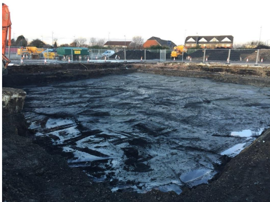
Plate 8: Excavation Area 2 looking north – large area of upper alluvium [160]
