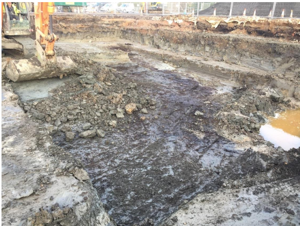
Plate 9: Excavation Area 2 looking north – revealing the peat [162]
