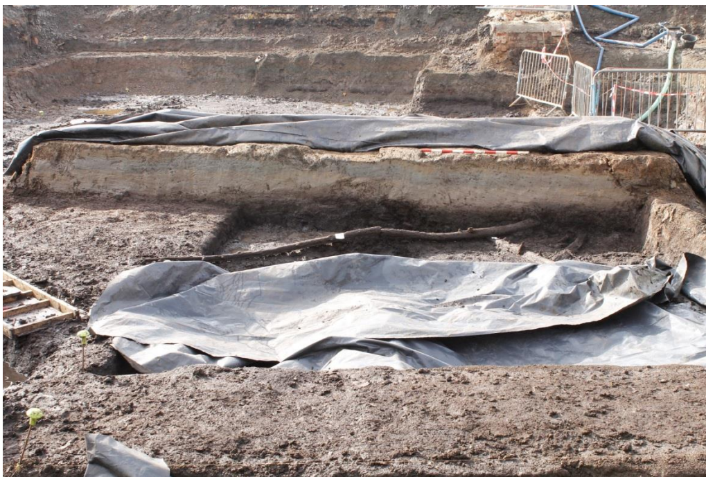
Plate 17: Excavation Area 3. Section 61 looking south
