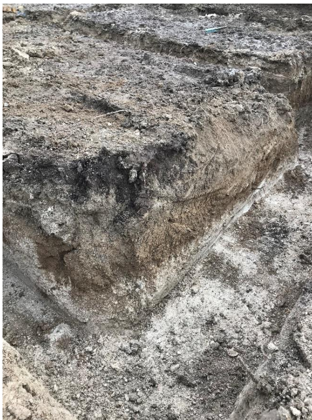
Plate 7: Foundation trench showing superficial head clay, Plot 2. Looking south-east.
