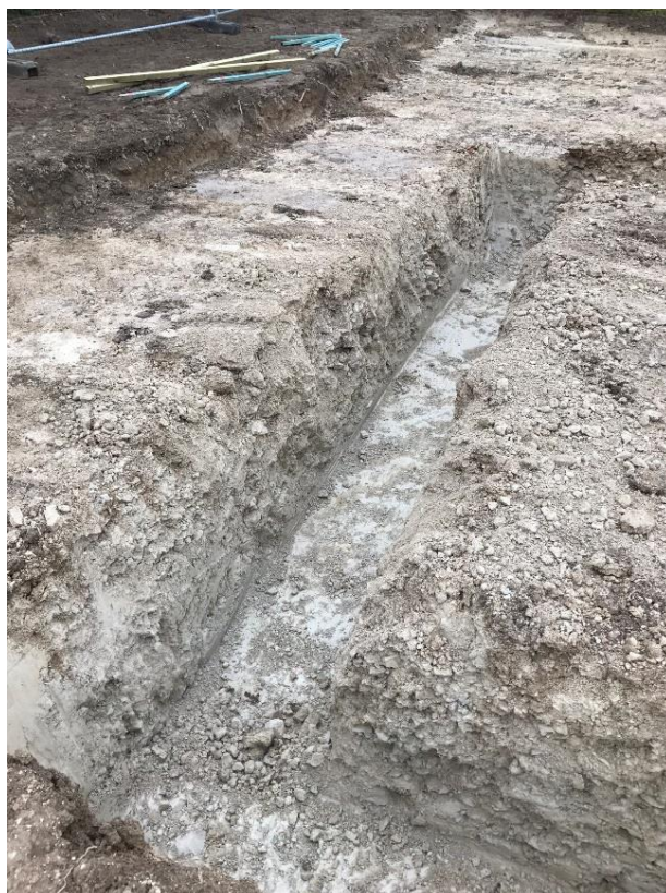
Plate 2: Foundation trench showing the natural chalk, Plot 3, Looking north-east.
