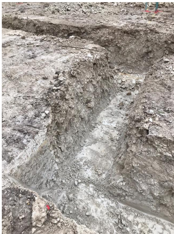
Plate 3: Foundation trench showing consolidated and loose chalk fragments, Plot 3. Looking east.
