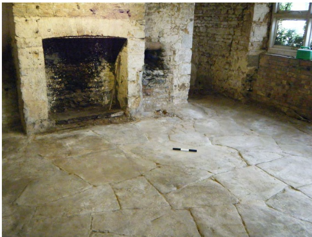
Plate 10: Flagstone floor in northern room of 37 West Street, looking SSW
