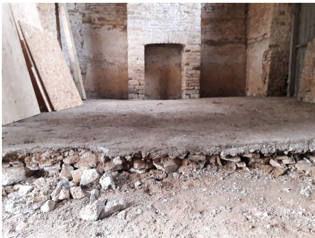
Plate 6: Ground reduction inside front barn, looking N
