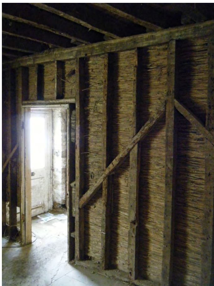
Plate 8: Reed Wall on ground floor
