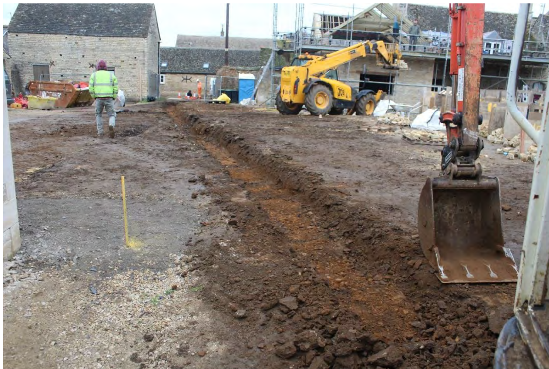
Plate 7: Service trench, looking E
