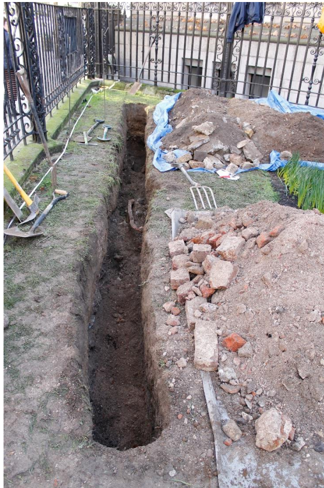
Plate 1: General view of trench, looking south-east
