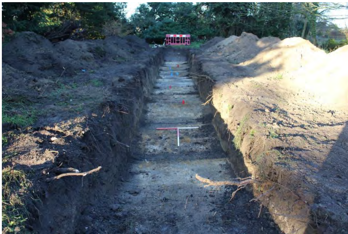
Plate 1: Pre-excitation shot of Trench 1 - looking East
