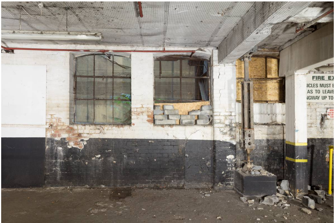
Plate 11 Lower ground floor level, windows to light well, looking east
