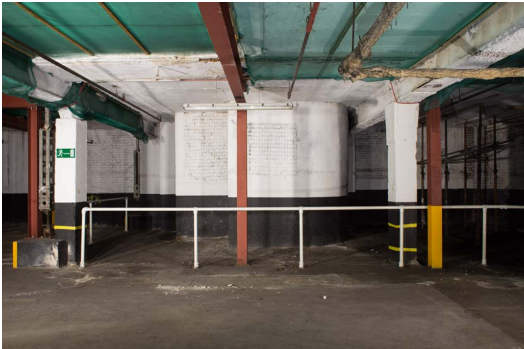
Plate 17c Lower ground floor level, western bays, looking west
