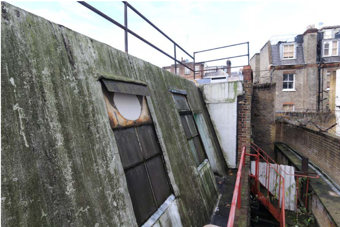
Plate 44 Roof level, detail of Mansard, looking north
