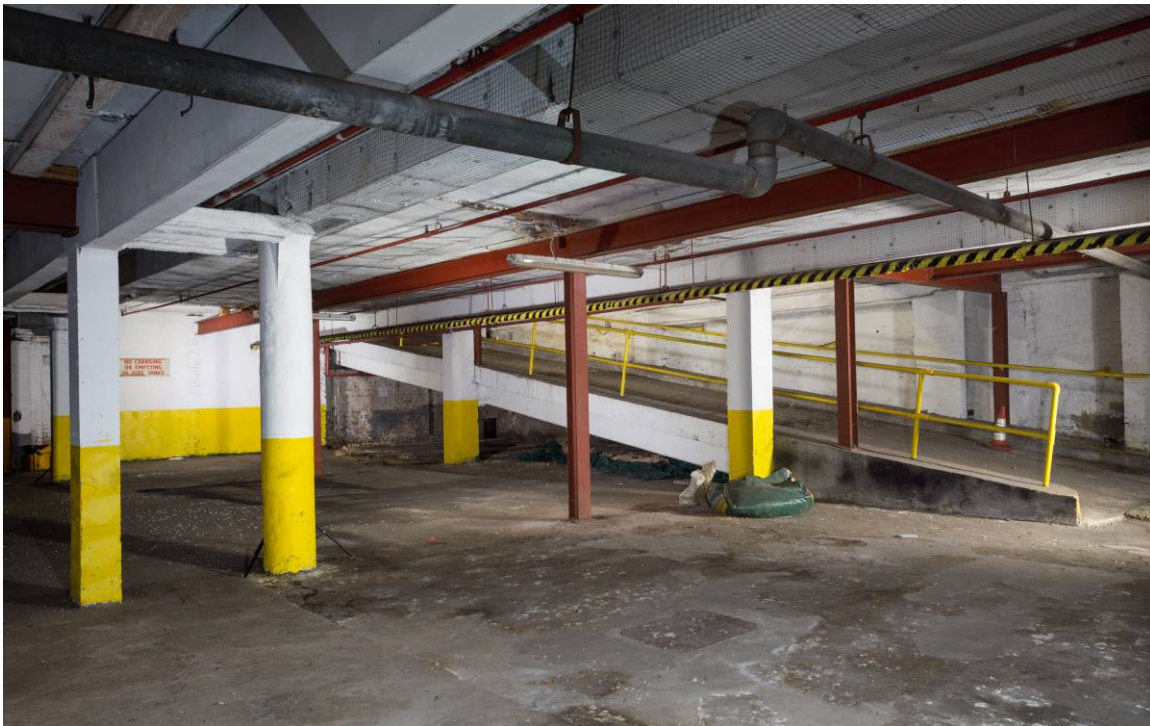
Plate 15 Lower ground floor level, central bays looking north-west towards ramp
