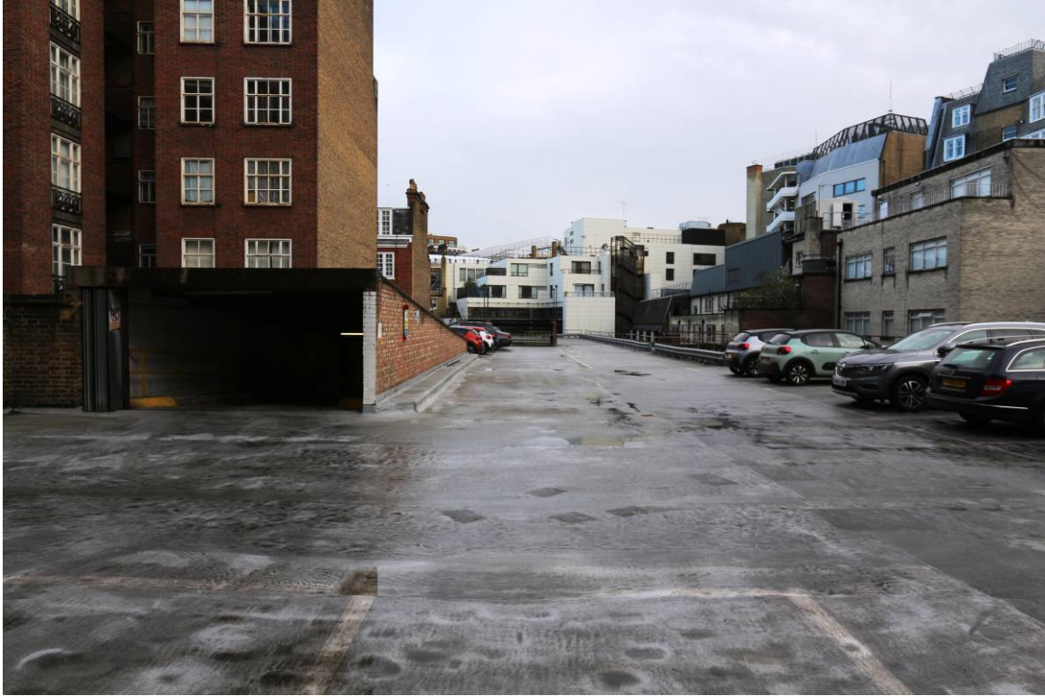
Plate 41 Roof level looking east
