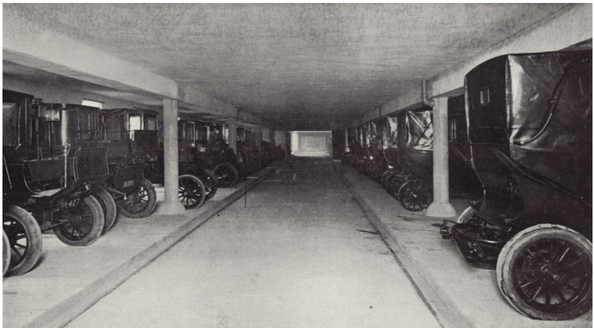
Historic Plate 6: First floor parking: note the runners for the transversers in the floor, looking west (The Car, 4 Dec 1907, 146)
