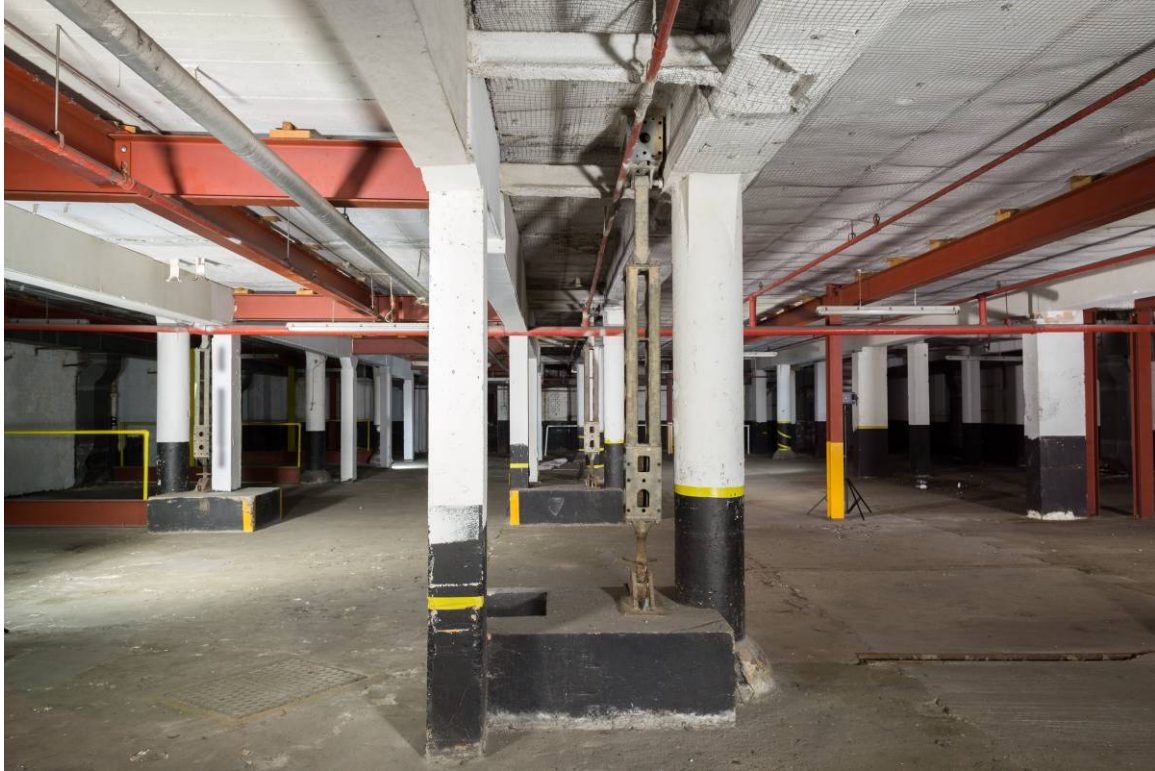
Plate10 Lower ground floor level, eastern bays, looking west
