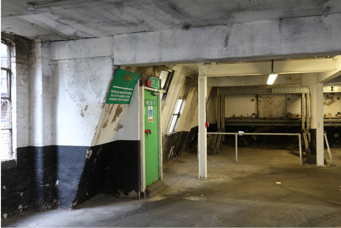
Plate 29 First Floor, eastern bays, return of Mansard roof looking south
