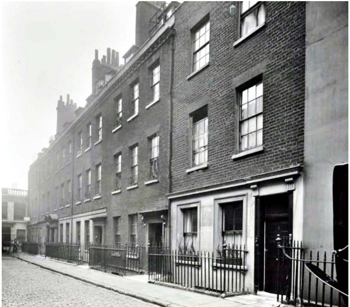
Historic Plate 9: Photograph taken in 1911 of Carrington Street with the entrance to the Electromobile Garage (far left)
