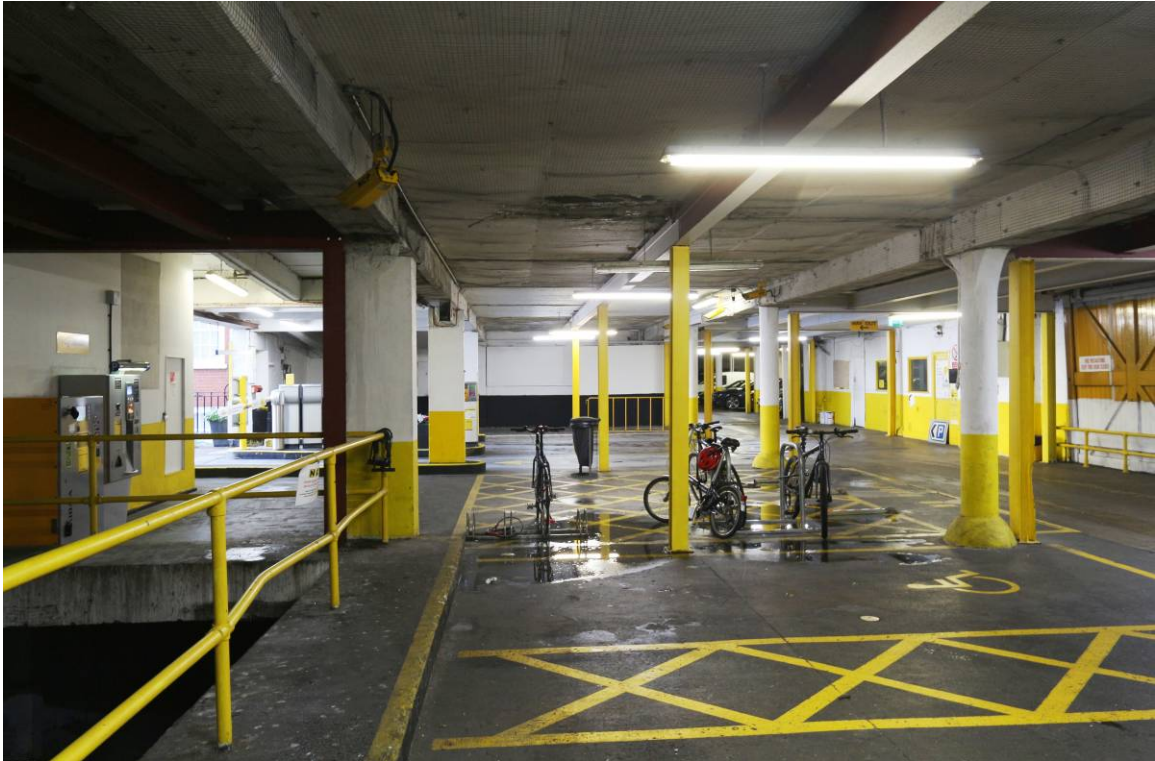
Plate 22 Upper ground floor level, central bay looking east
