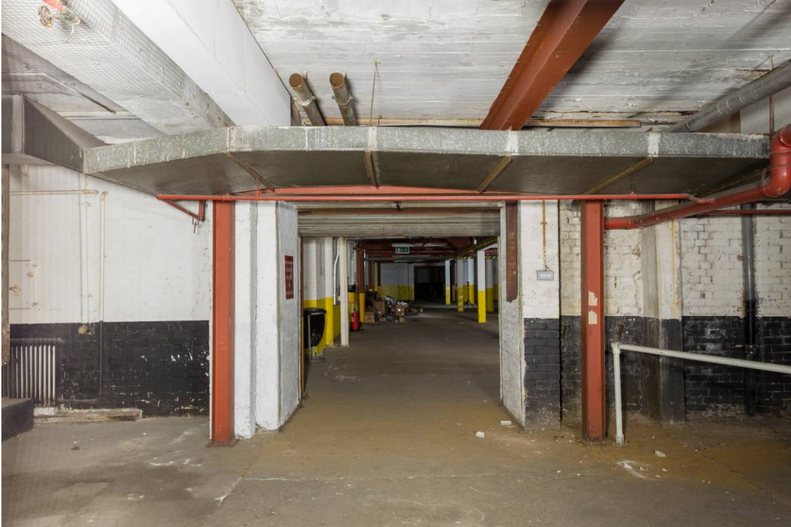
Plate 12 Lower ground floor level, looking west to central bays
