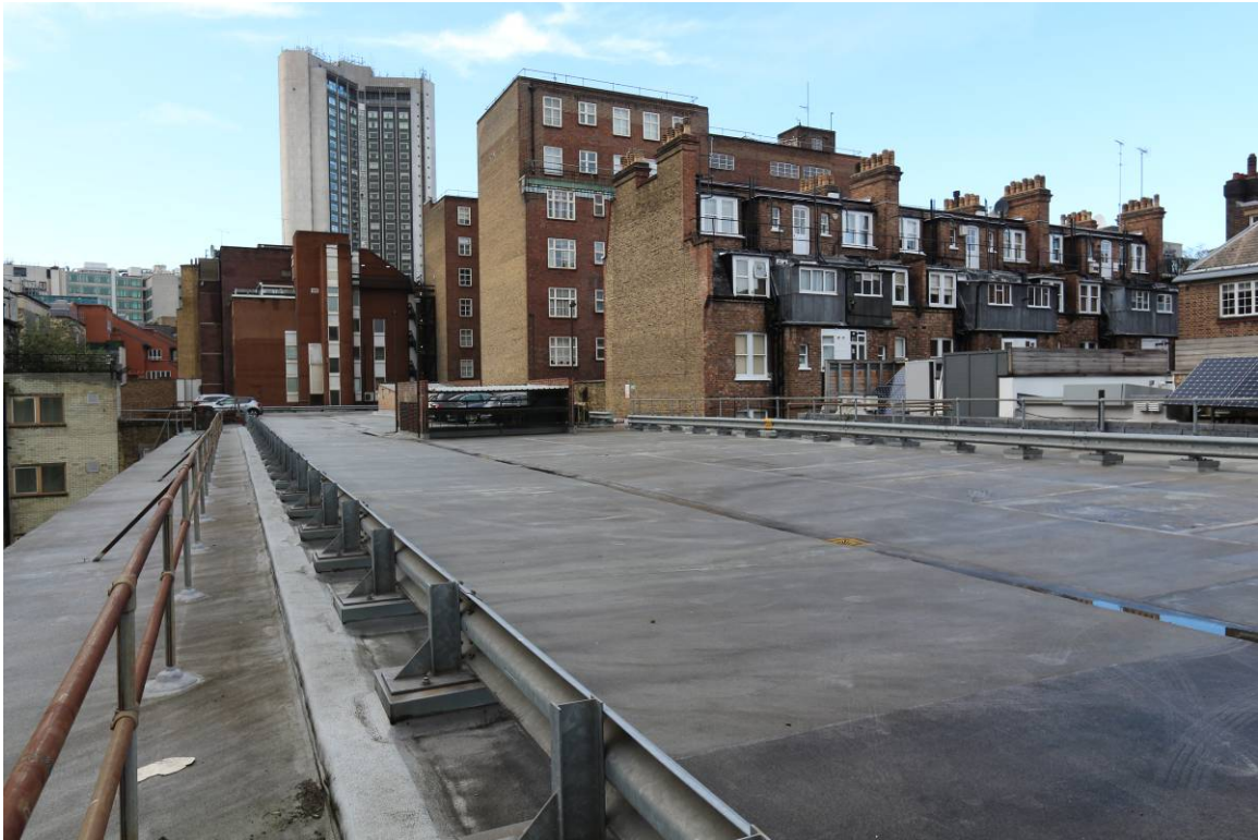
Plate 42 Roof level looking west
