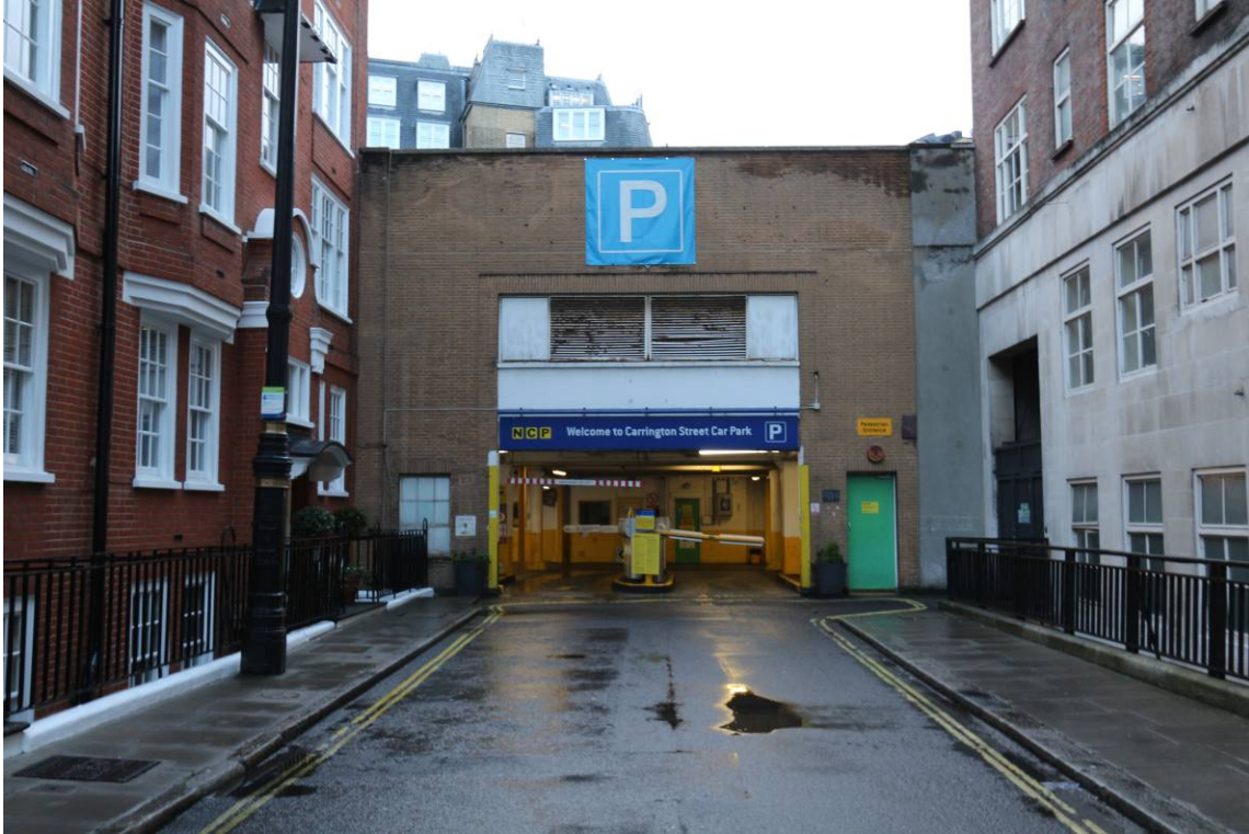
Plate 1 View from Carrington Street Looking south, showing rebuilt façade
