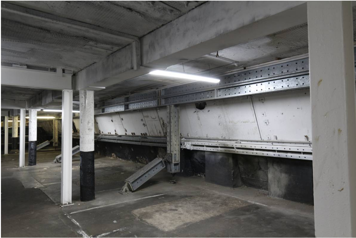
Plate 28 First Floor, eastern bays, structural props
