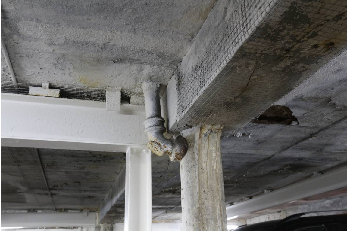
Plate 37 First Floor, eastern bays, column with integral drain
