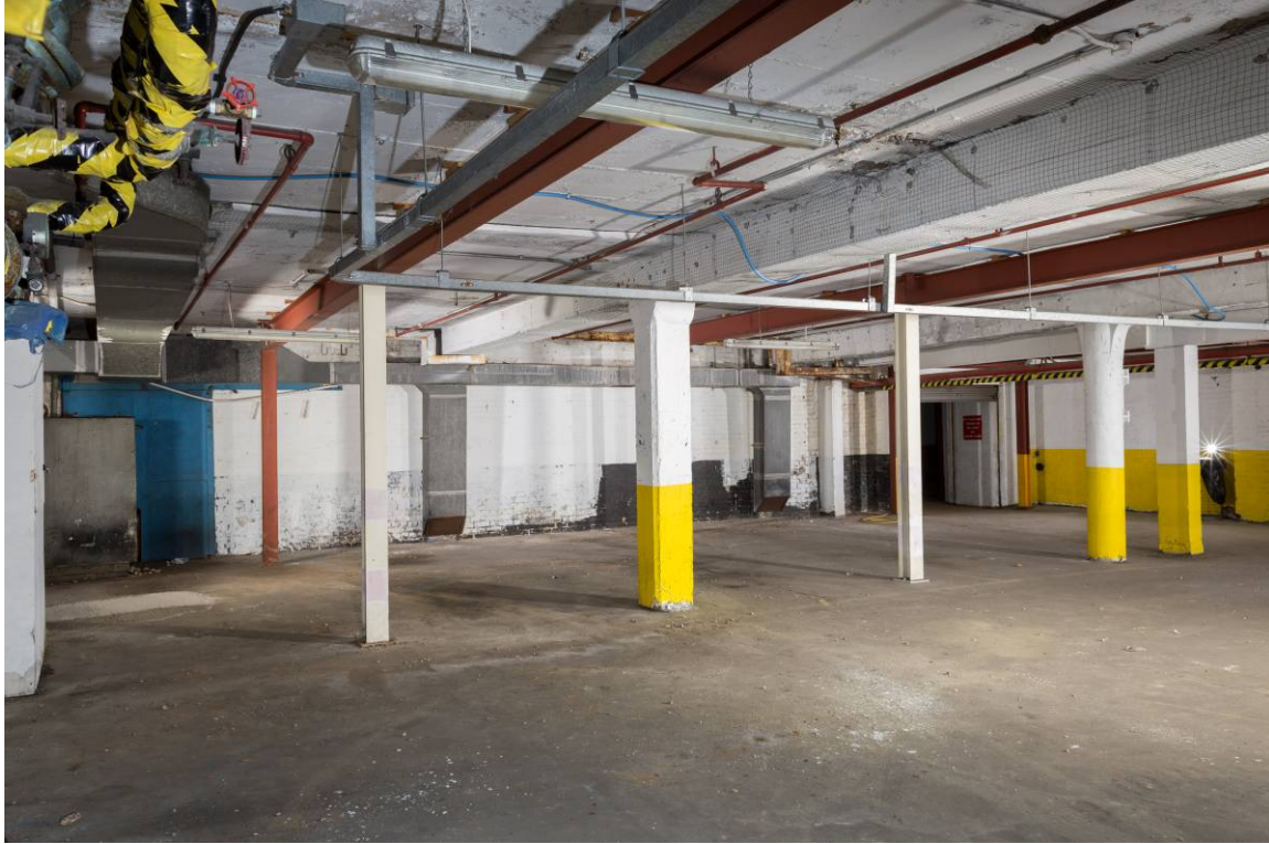
Plate 14 Lower ground floor level, central bays, looking south-east
