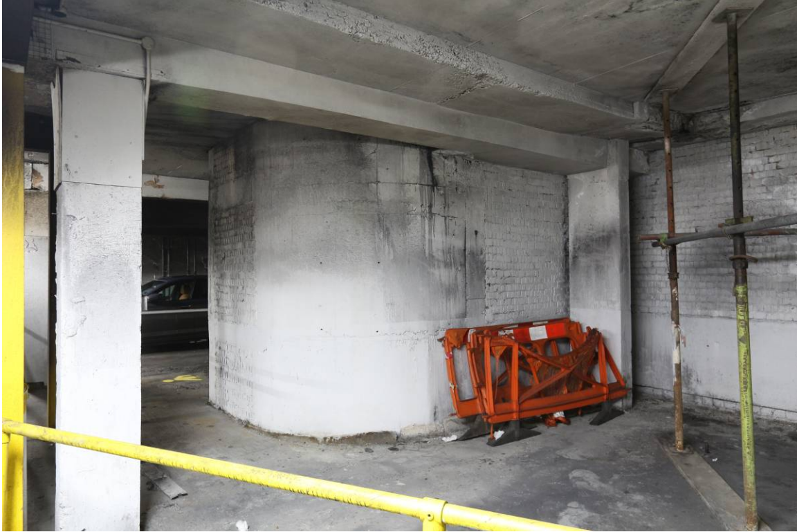
Plate 27 Upper ground floor level, western bays, looking toward stairwell
