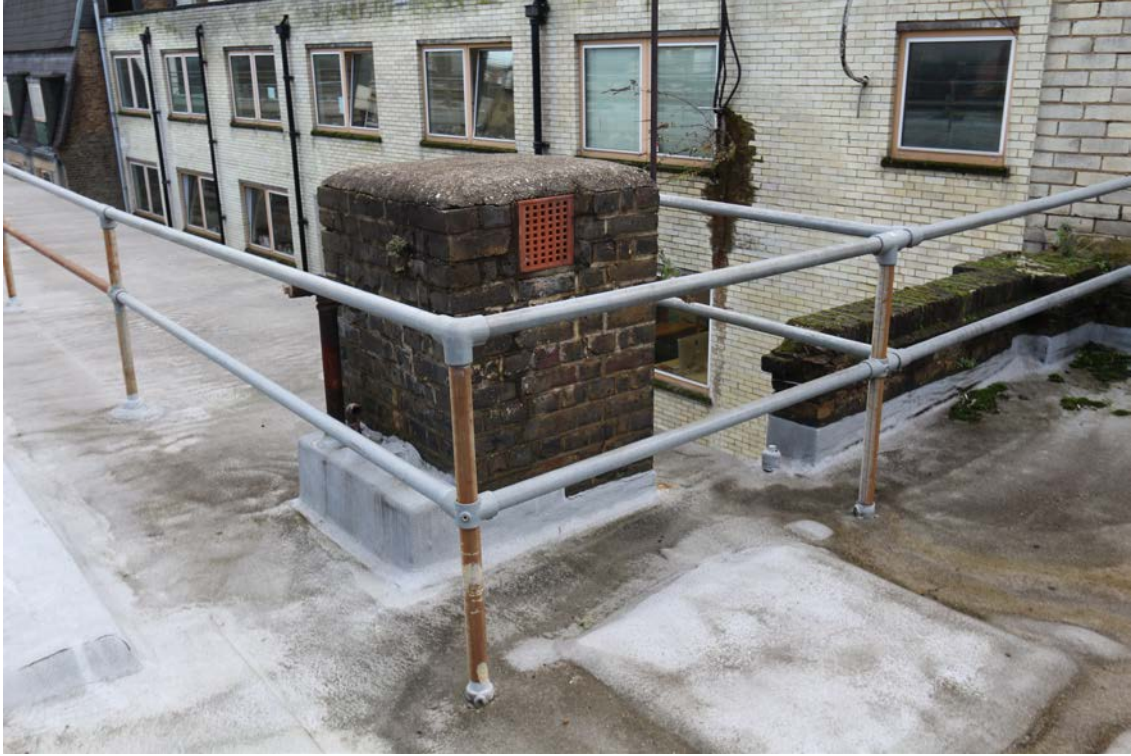
Plate 45 Roof level, chimney, looking south-east
