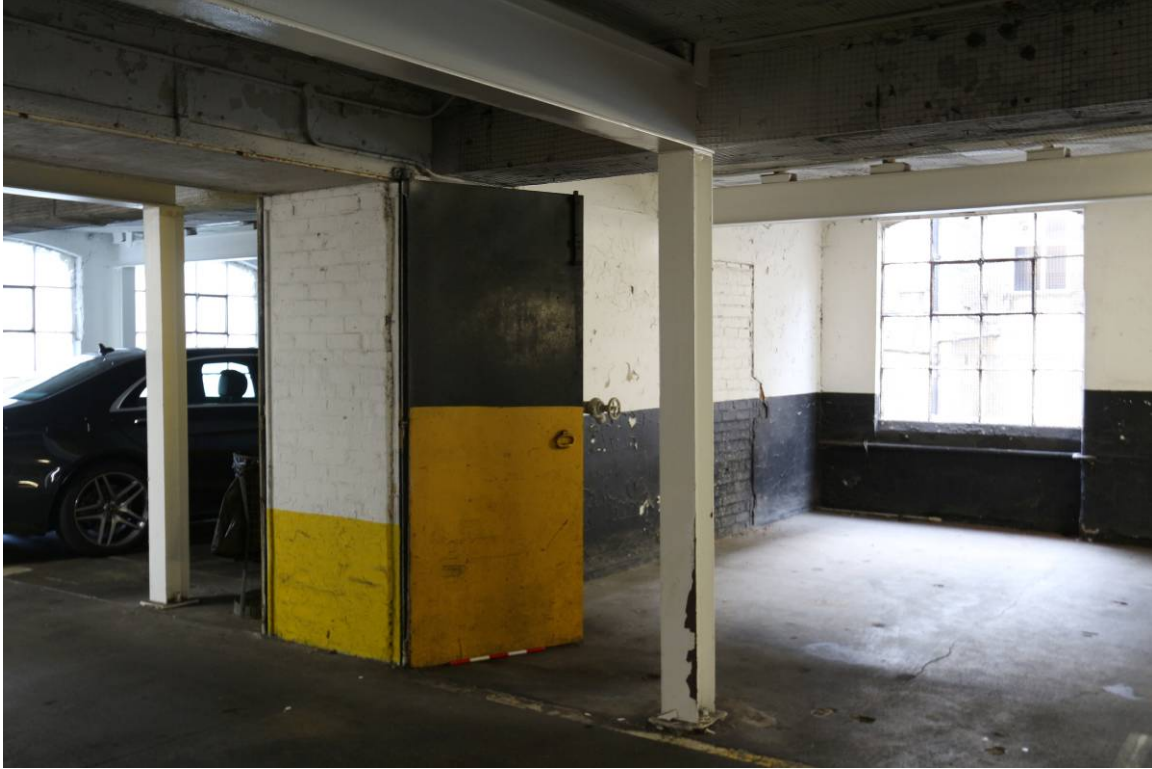
Plate 32 First Floor, western bays, steel fire/security door
