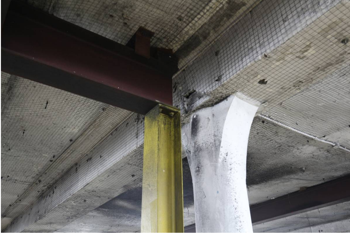
Plate 8 Typical column head and later steelwork on the first floor
