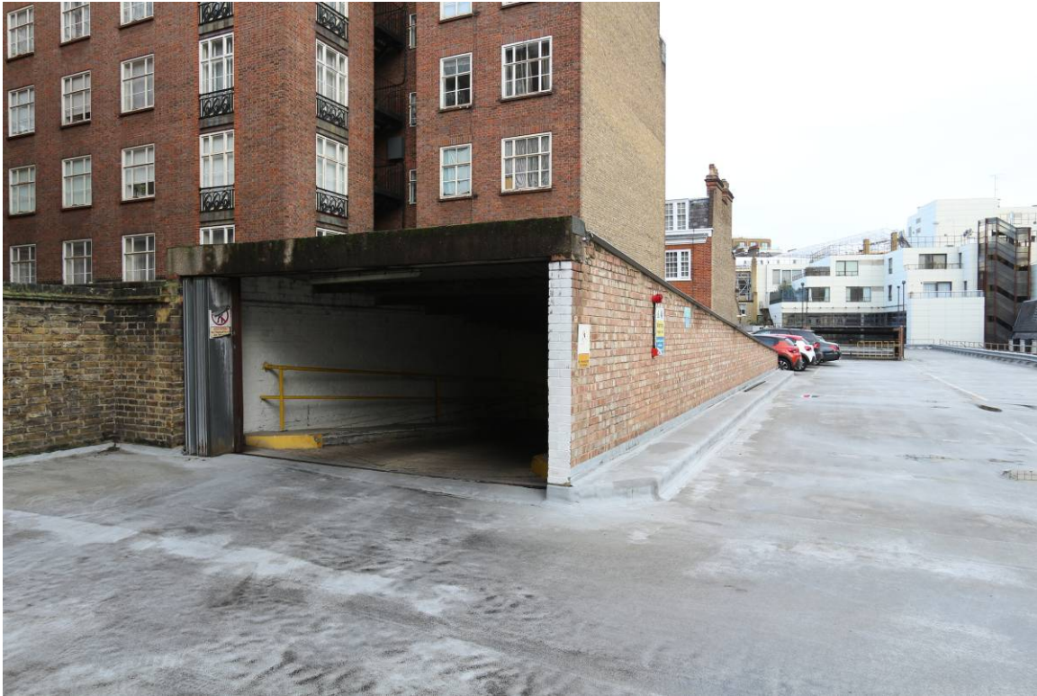
Plate 40 Ramp up onto roof level, looking east
