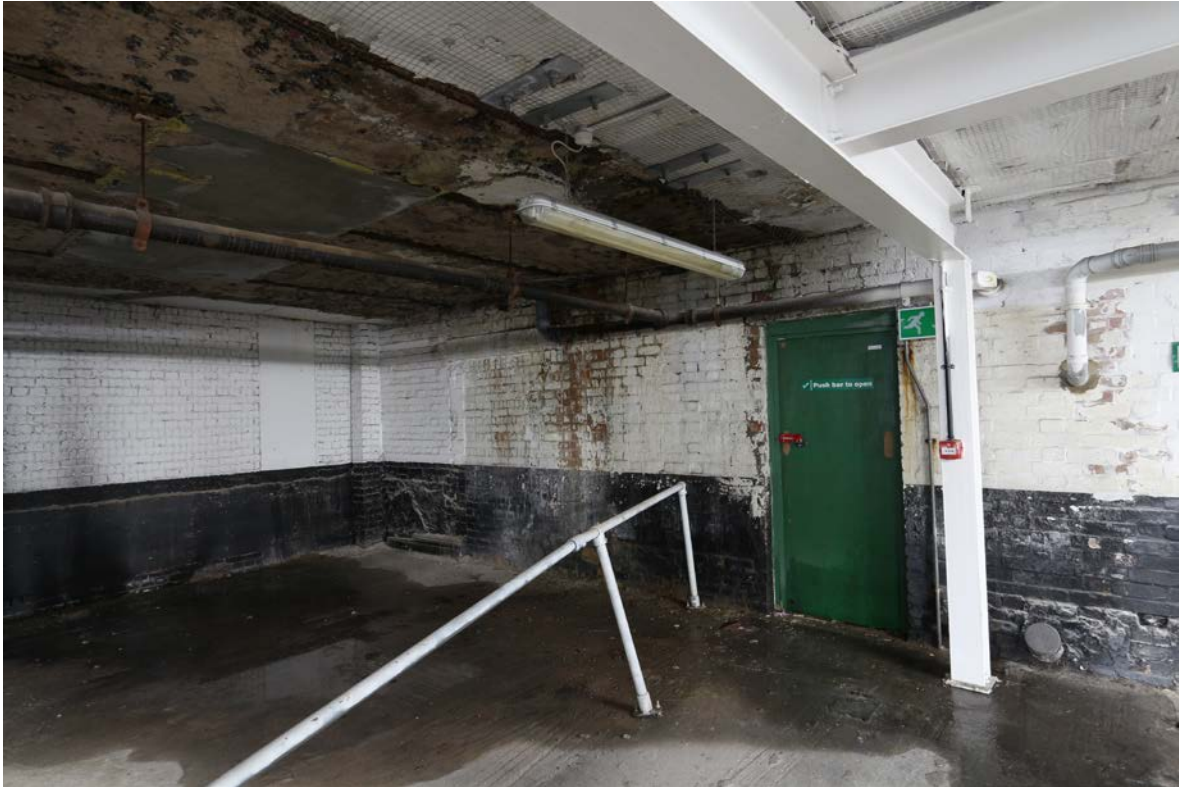
Plate 33c First Floor, western bays, looking north-west
