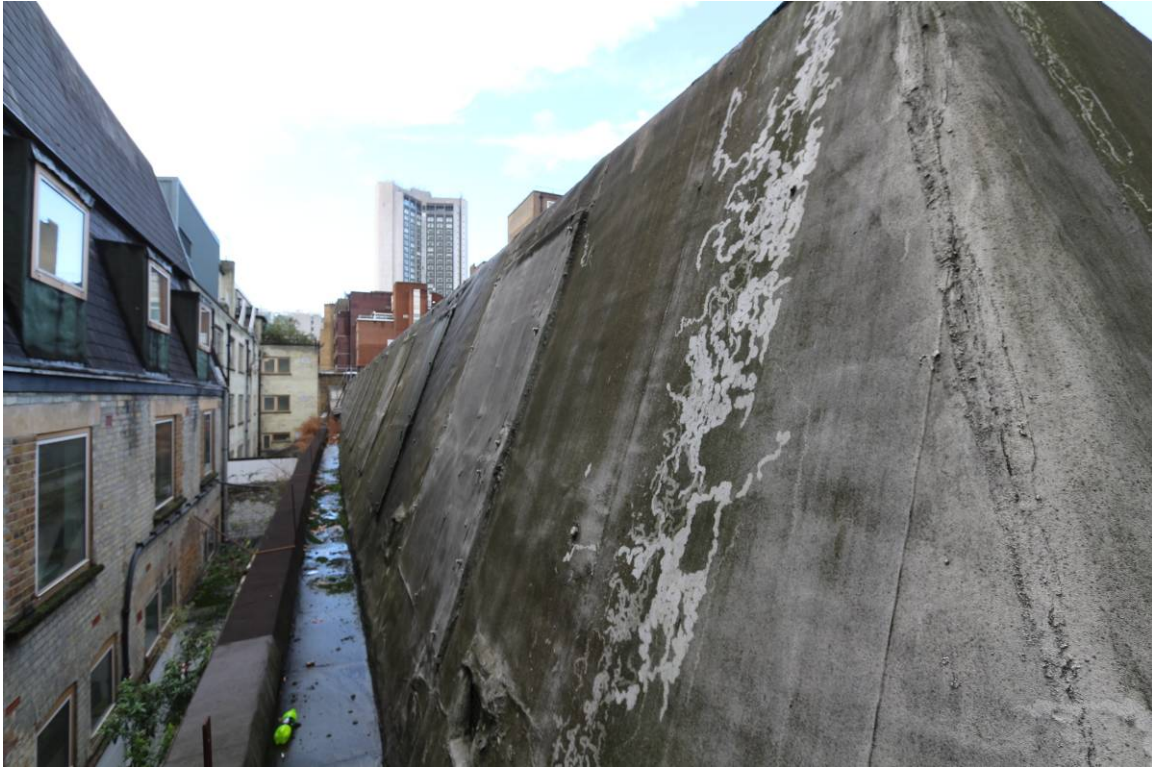
Plate 43 Roof level, detail of Mansard, looking west
