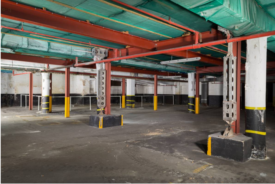
Plate 18 Lower ground floor level, western bays, looking north-east
