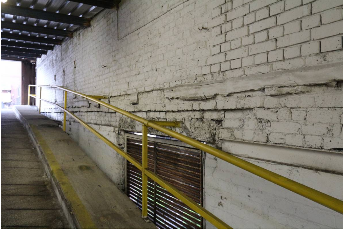
Plate 39 First Floor, wall scar of former ceiling/roof structure
