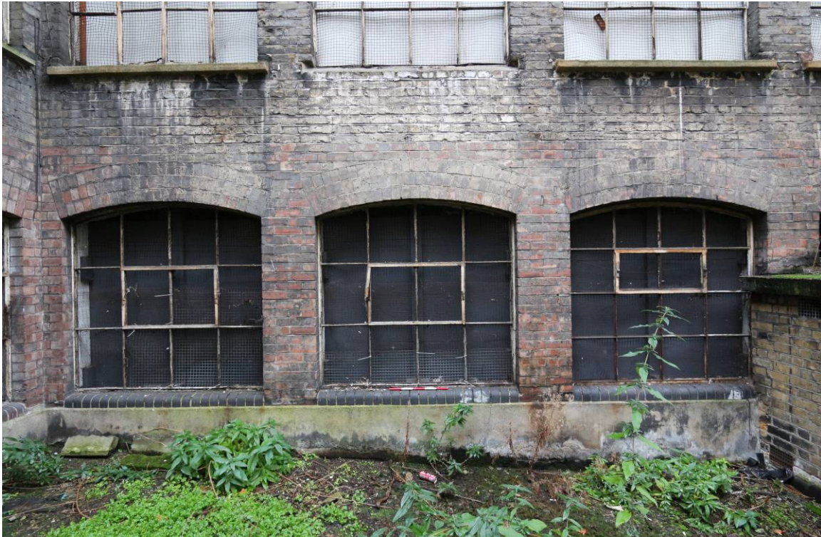
Plate 4 Detail of Lower Ground windows
