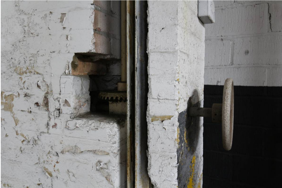
Plate 31 First Floor, eastern/central bays, detail of hand-operated shutter door mechanism
