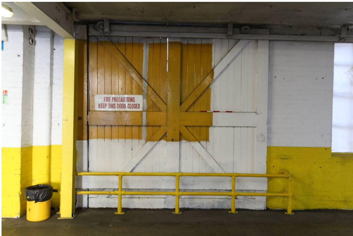
Plate 24 Upper ground floor level, central bays, former doorway into rear yard
