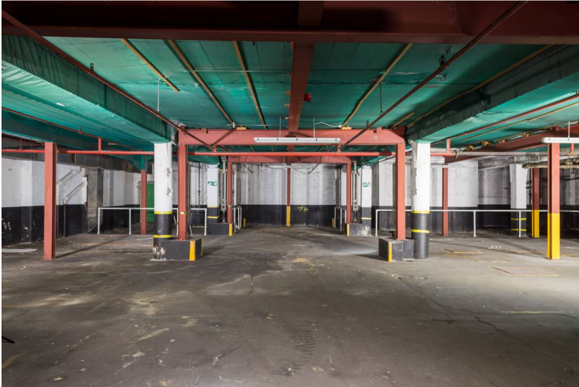
Plate 17a Lower ground floor level, western bays, looking west
