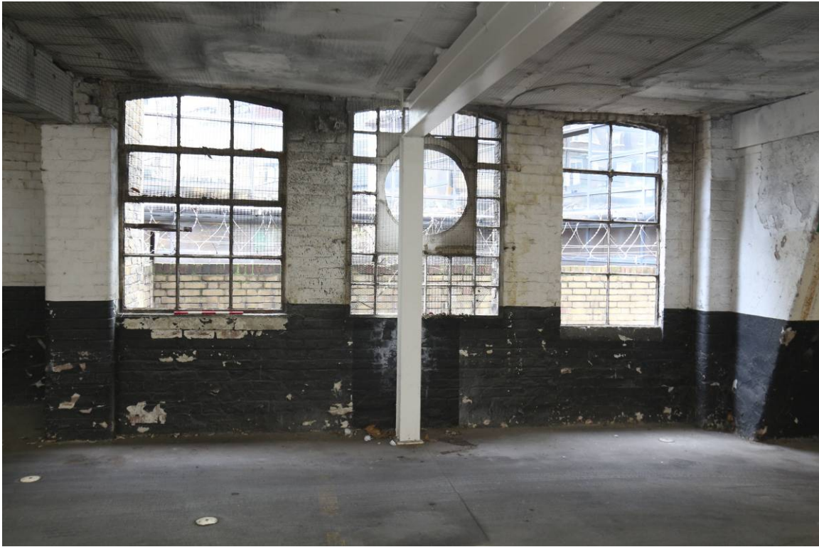
Plate 30a First Floor, eastern bays, windows
