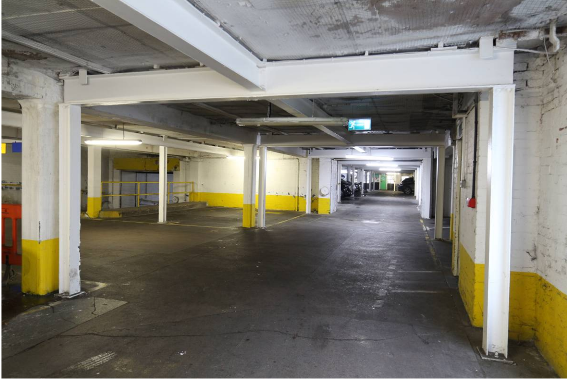
Plate 35 First Floor, central bays, looking east
