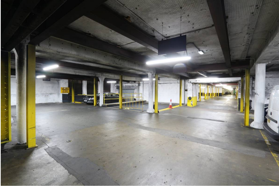
Plate 25a Upper ground floor level, western bays, looking north-east
