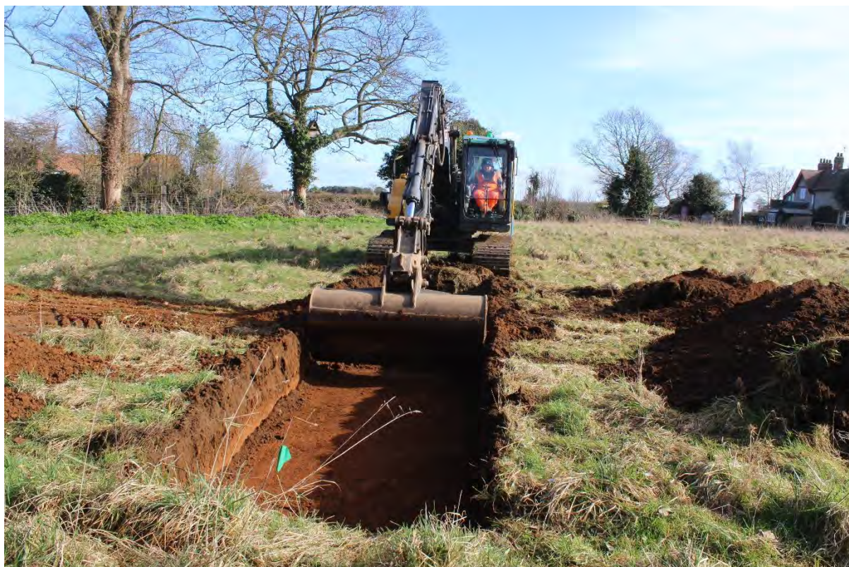
Plate 2: 14 tonne 360° Excavator opening an evaluation trench
