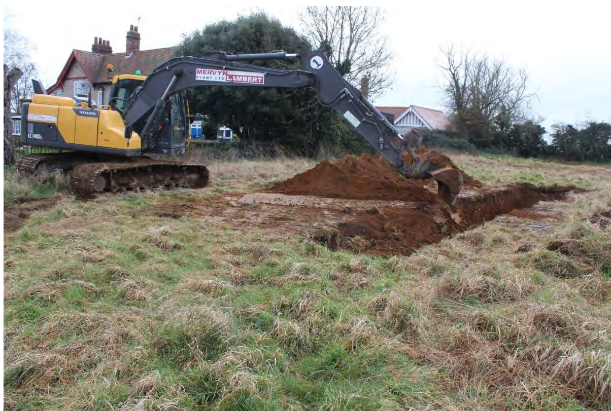
Plate 16: Backfilling the trenches with the excavator
