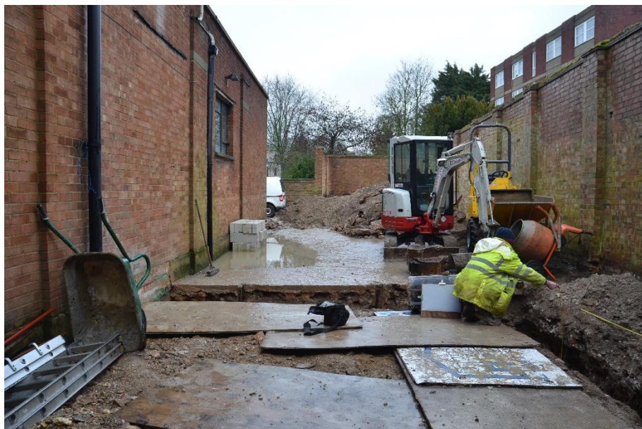
Plate 1: Site view northeast
