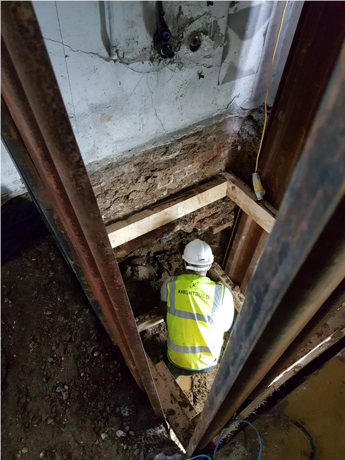
Plate 1: North-east facing view of underpinning in Excavation Pit 1.
