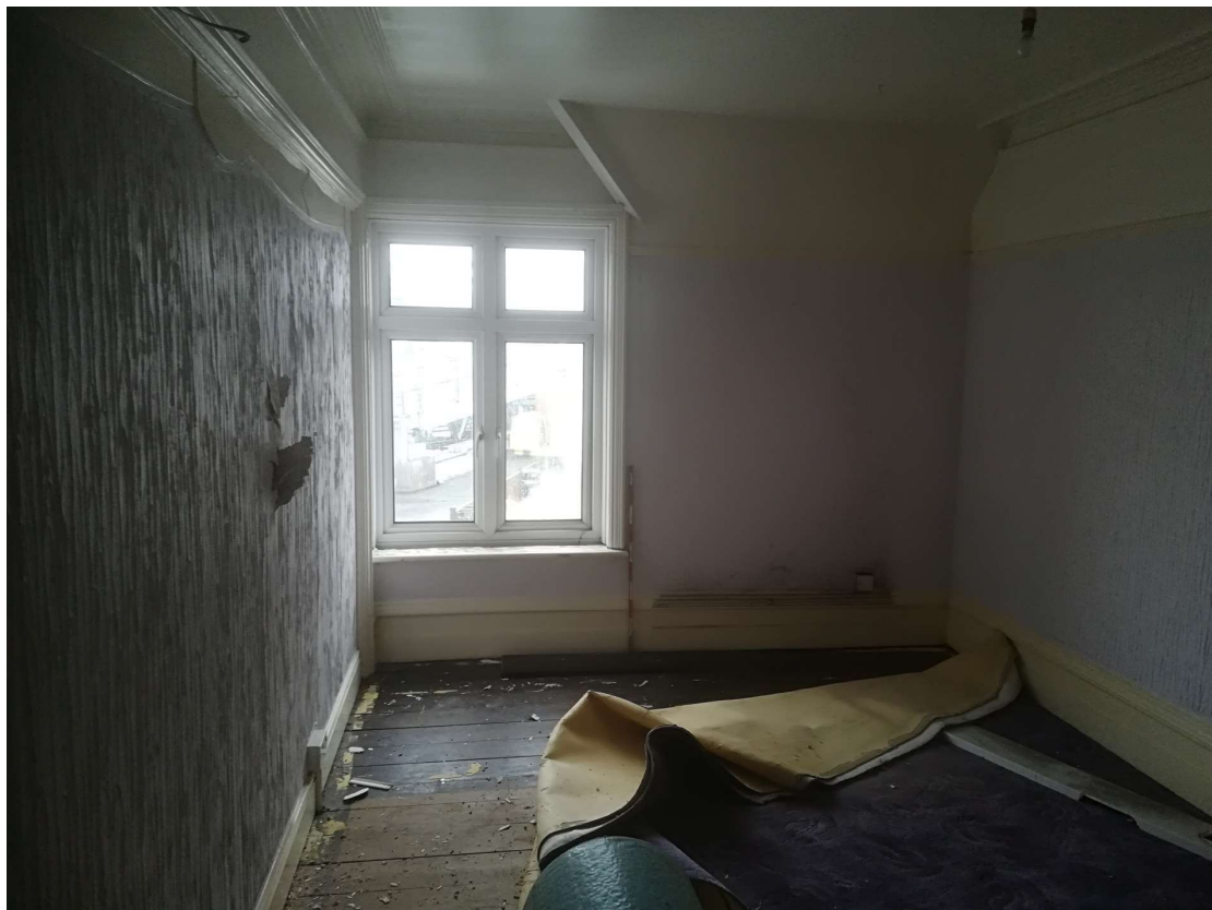
Plate 20. Room 10: Upper storey bedroom, looking north. Scale 1m.
