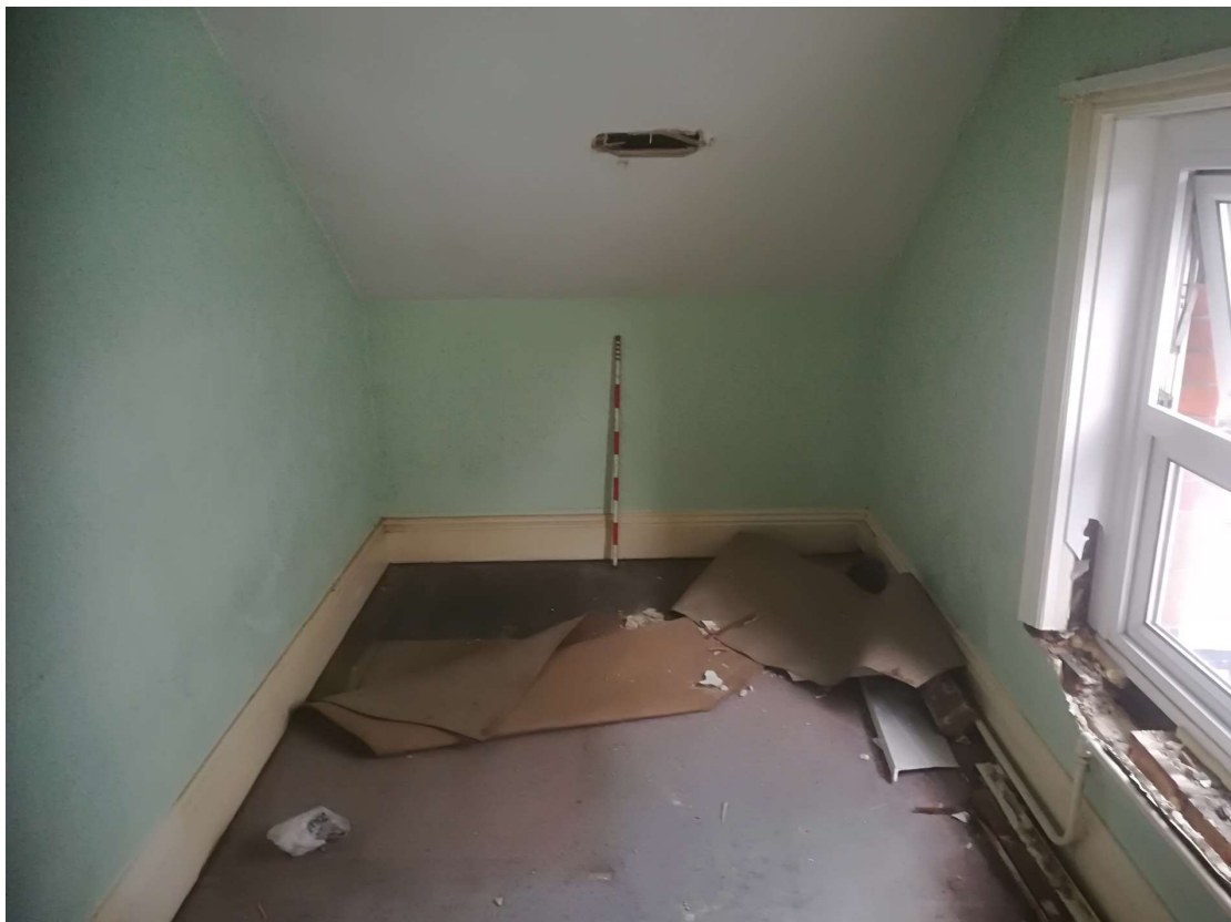
Plate 16. Room 6: Upper storey bedroom, looking north-east. Scale 1m.
