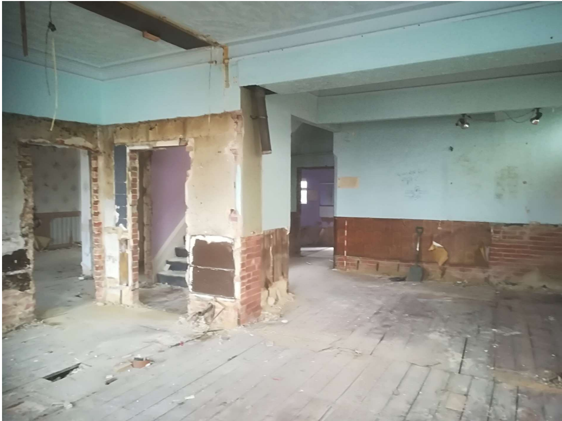
Plate 7. Room 1: Public bar looking north-east. Scale 1m.
