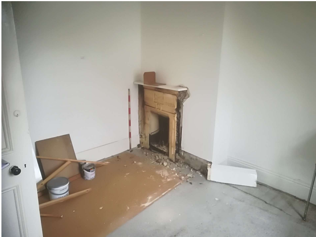
Plate 21. Room 12: Upper storey bedroom, looking north. Scale 1m.
