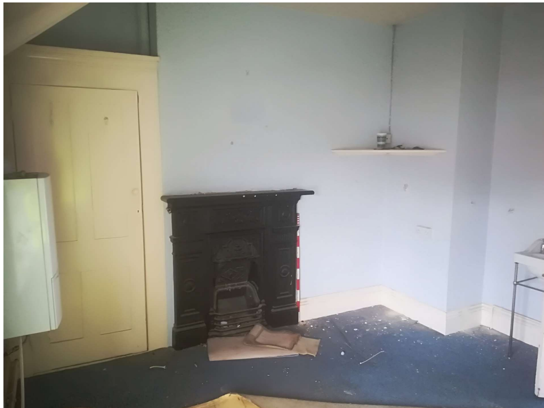
Plate 18. Room 8: Upper storey bedroom, looking north. Scale 1m.
