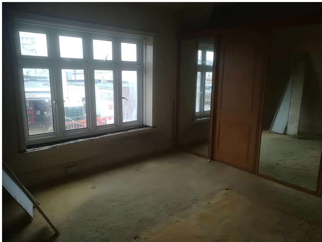
Plate 22. Room 11: Upper storey bedroom, looking east. Scale 1m.
