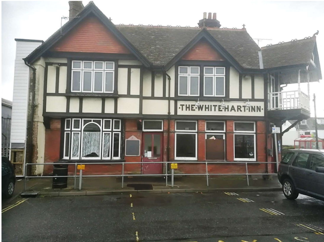
Plate 5. External west-facing elevation of the building. Scale 1m.
