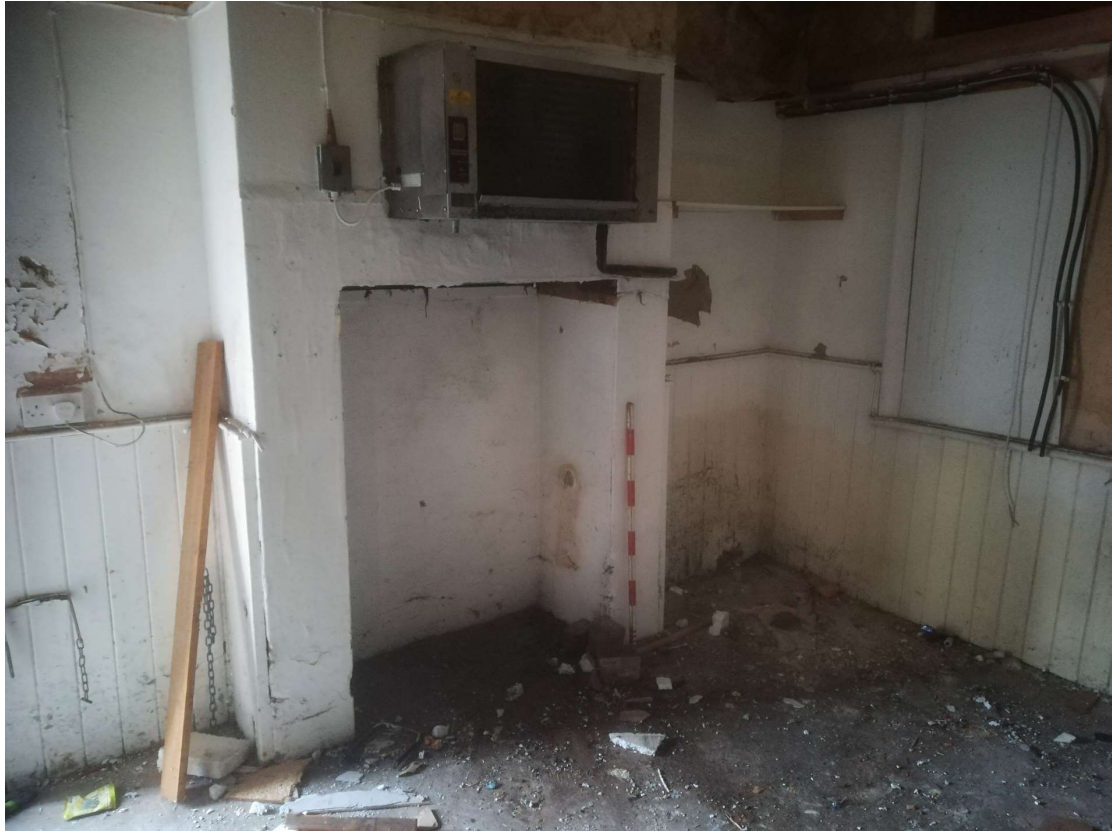
Plate 13. Room 5: Chimney breast looking south. Scale 1m.
