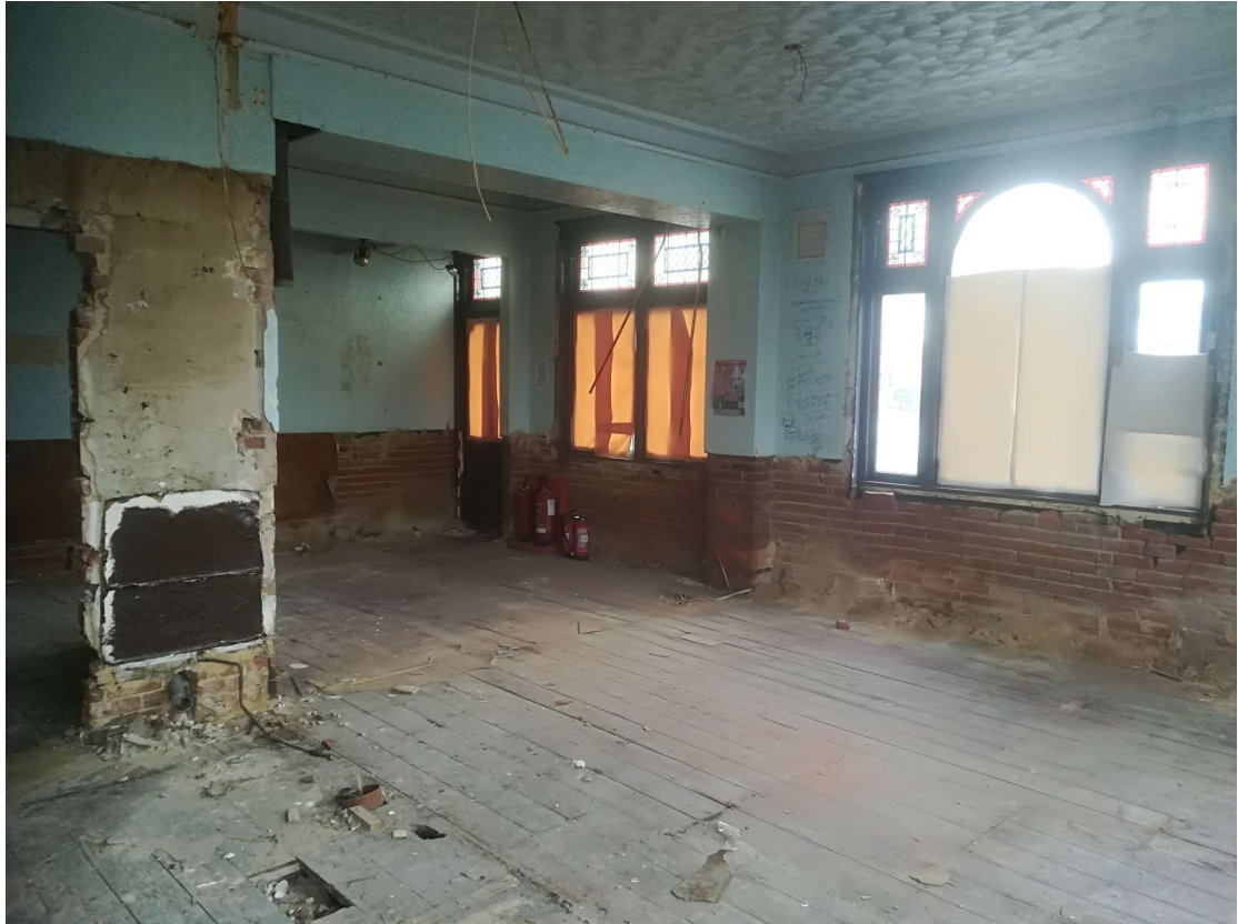
Plate 9. Room 1: Public Bar looking south-east. Scale 1m.
