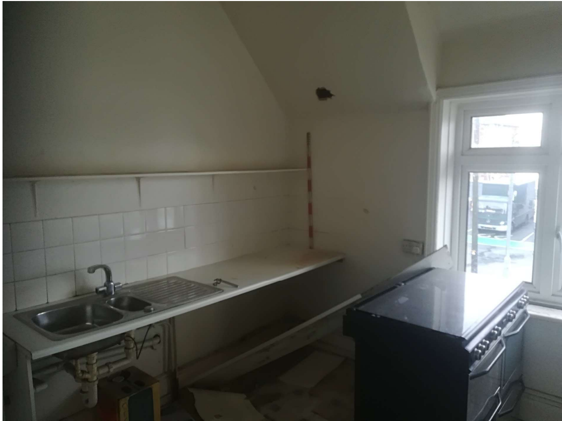
Plate 17. Room 7: Upper storey kitchen, looking south. Scale 1m.
