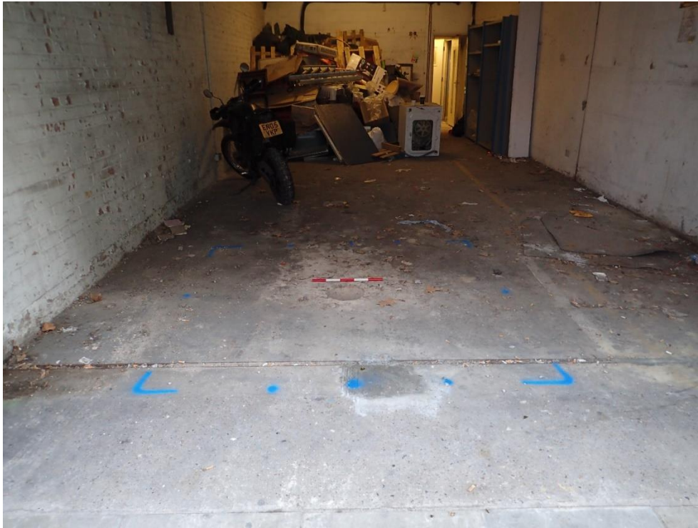
Plate 1: Garage with Borehole 1. Looking north.
