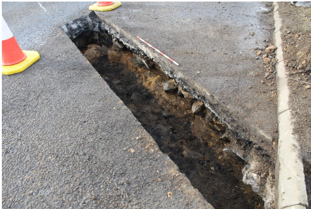
Plate 1: Overview of Trench 1 (SW-facing direction of view)
