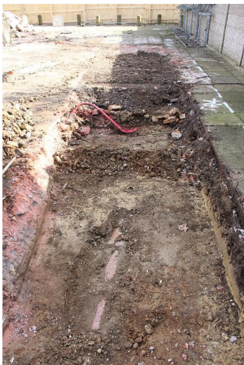
Plate 5: East view of Trench 4 showing buried services (1m scale).
