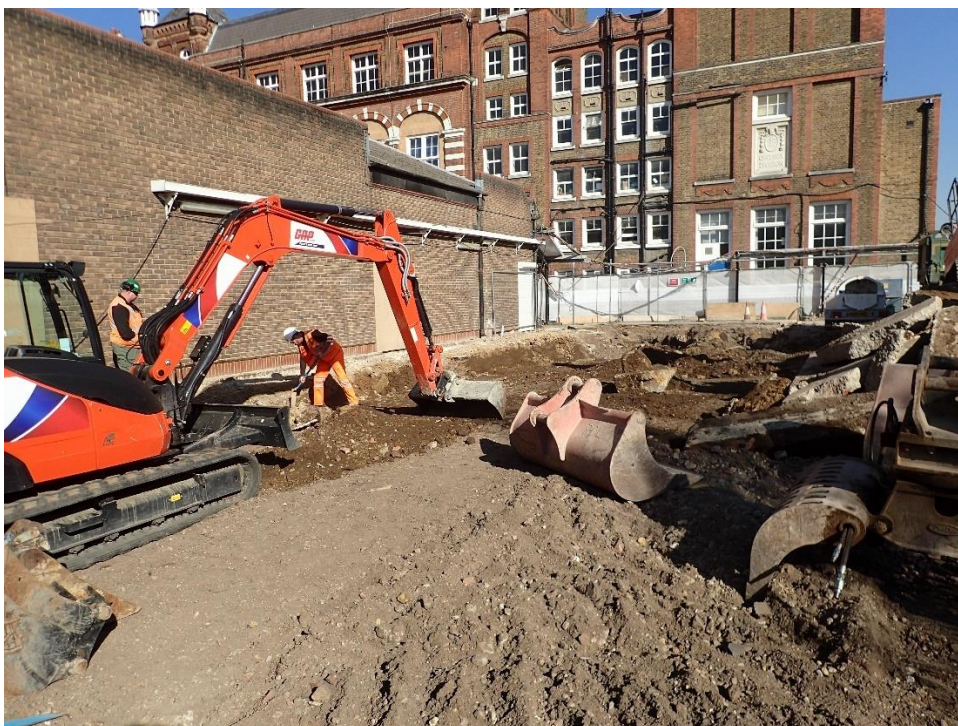
Plate 3: machine excavation of drain run, looking northeast.
