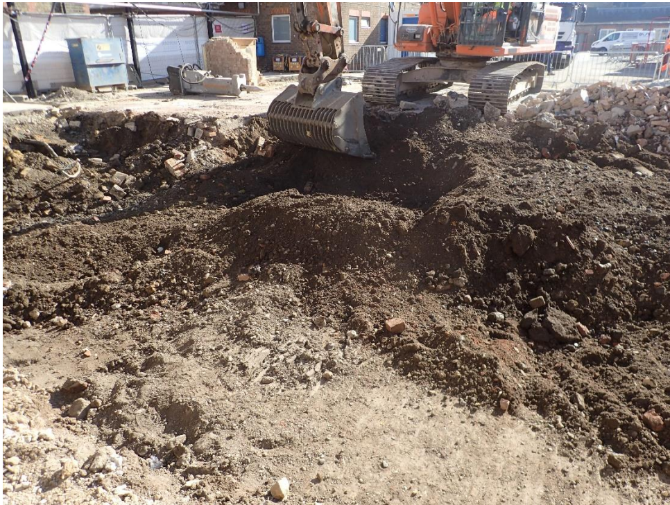
Plate 1: Area of obstruction removal, looking east.
