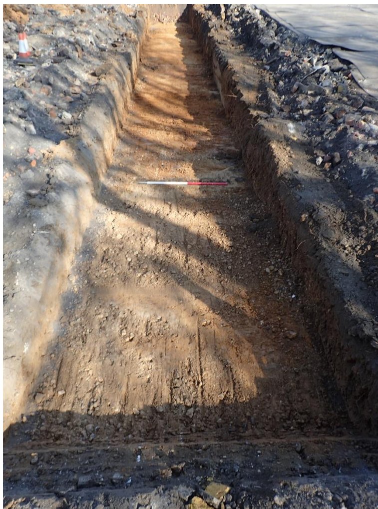
Plate 3: Trench 3, view to north, 1m scale
