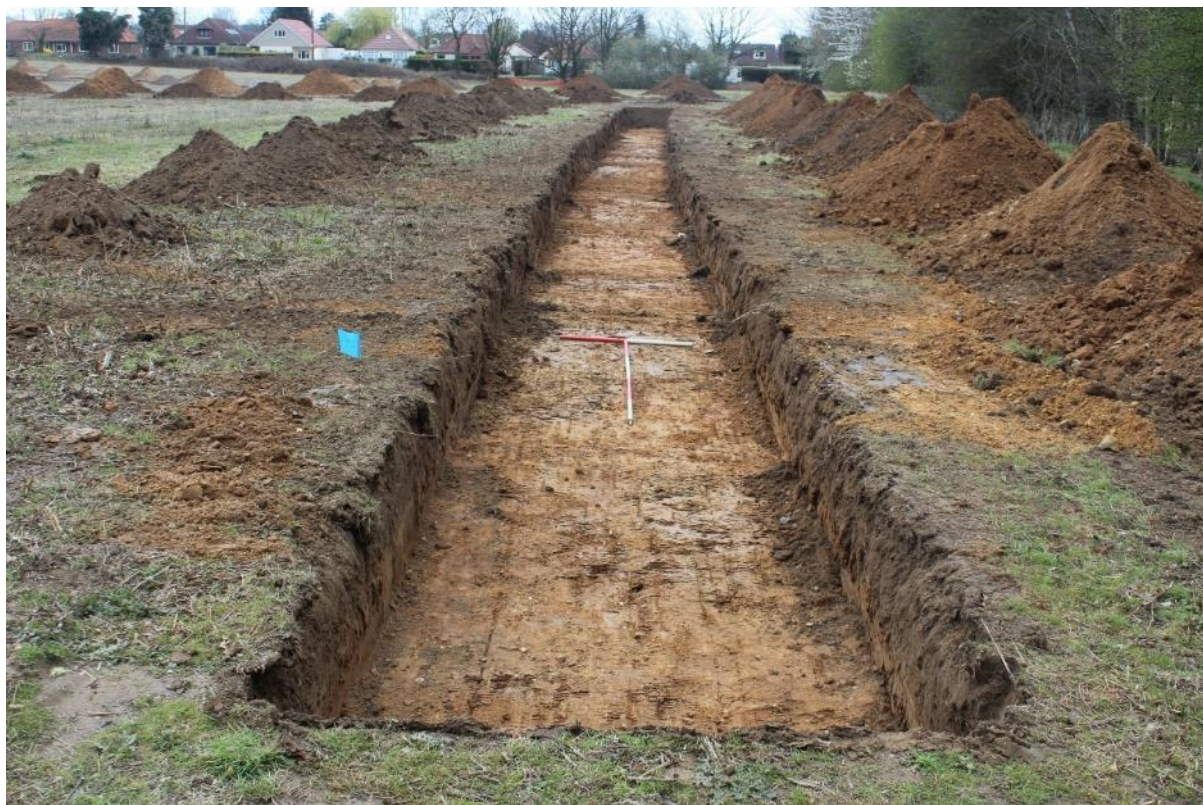
Plate 53 Northeast view of Trench 23
