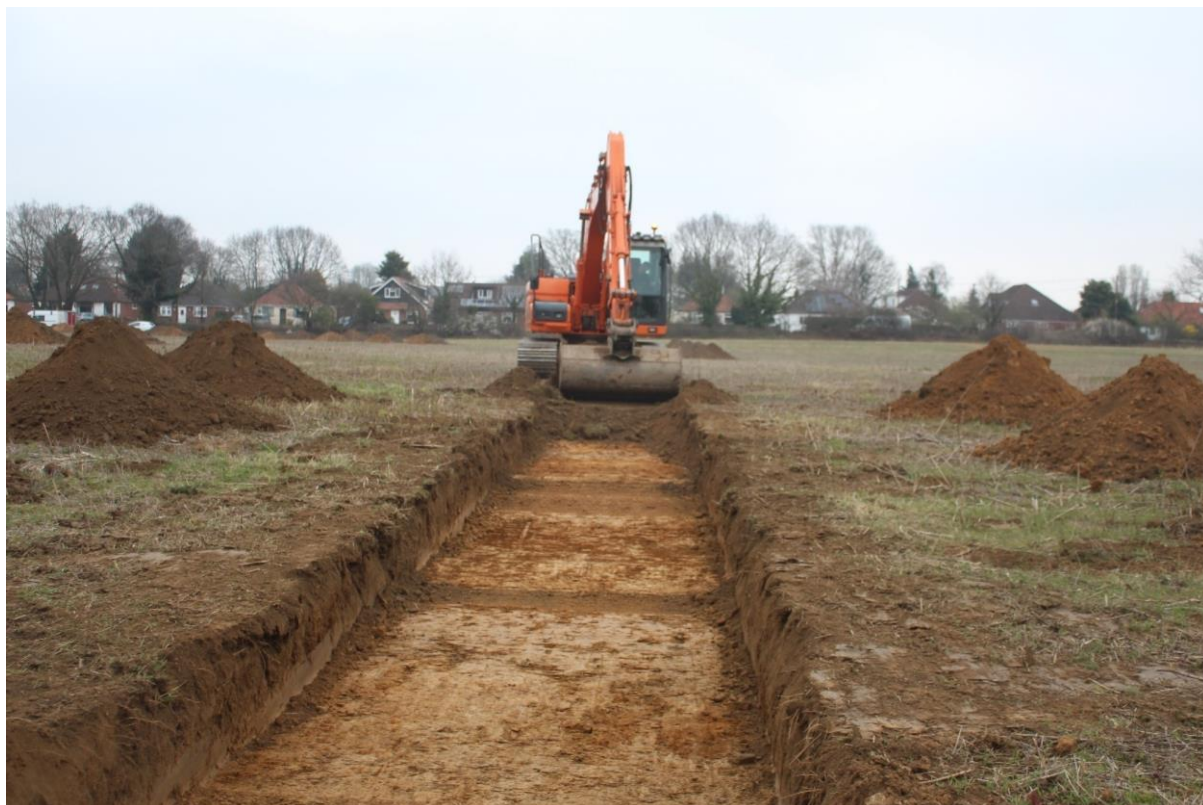
Plate 57 14-ton 360 Machining within Trench 6
