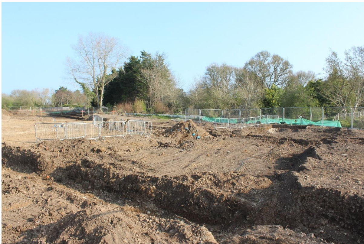
Plate 1. Shot of site facing northeast.
