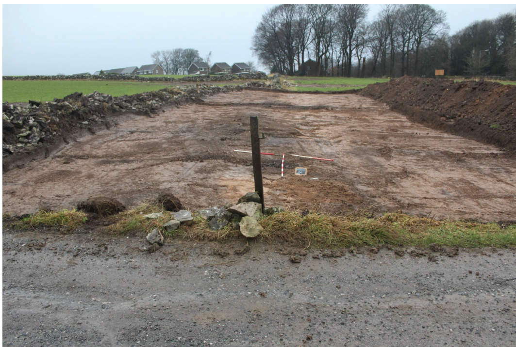
Plate 1: Shot of site looking northwest
