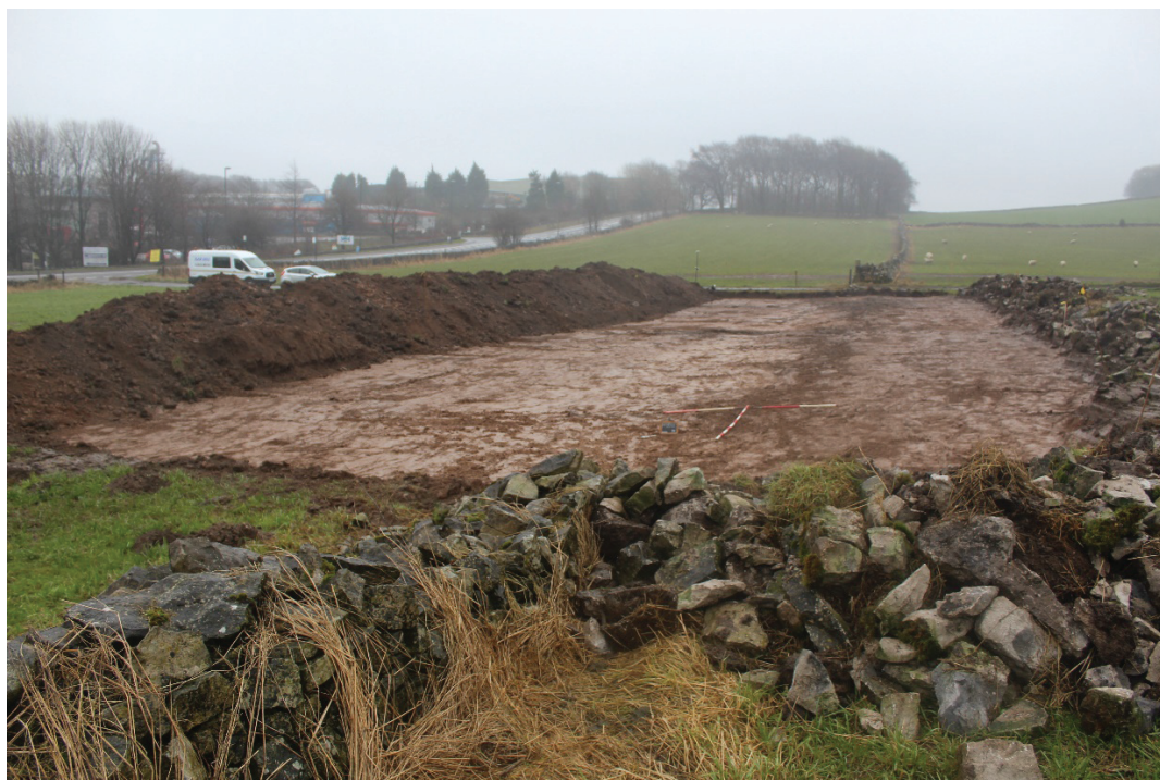
Plate 2: Shot of site looking southeast showing extant drystone wall
