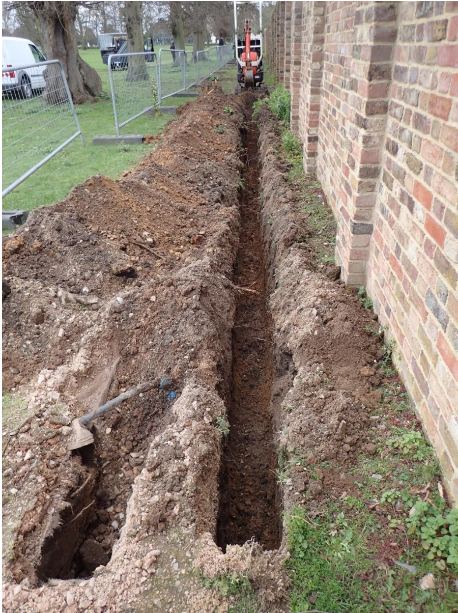
Plate 1: Irrigation Trench, facing west
