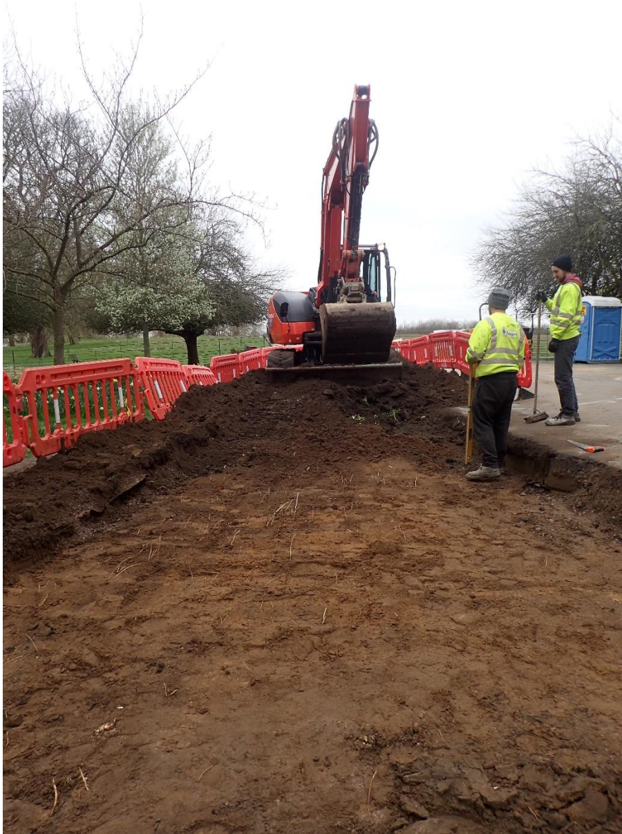
Plate 4: Road widening area facing southwest
