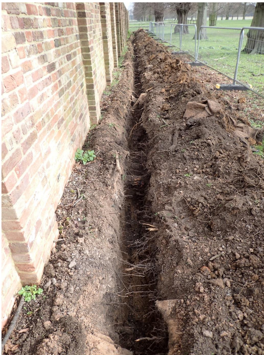
Plate 2: Irrigation Trench, facing east
