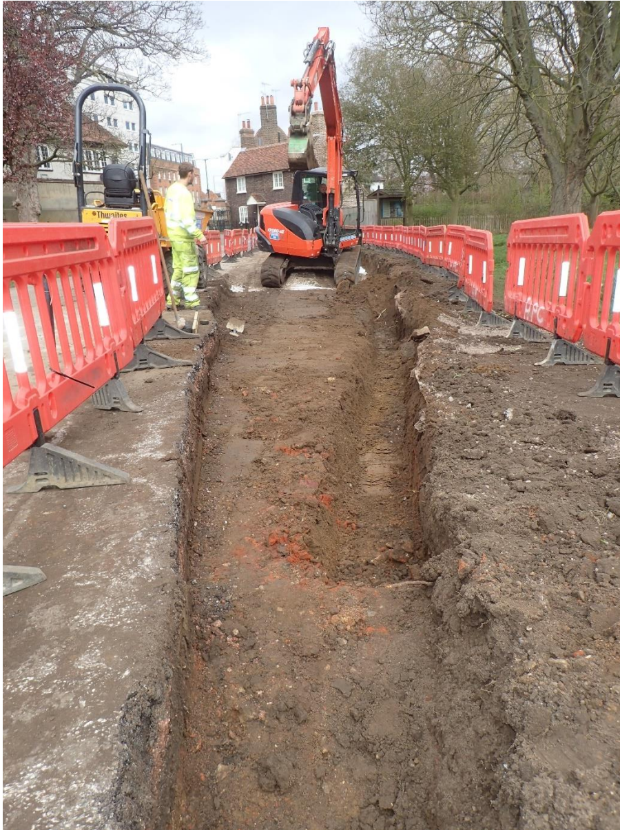
Plate 5: Road widening area facing northeast
