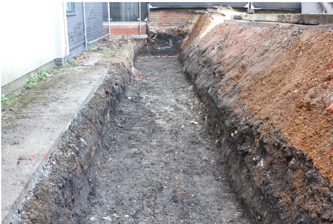
Plate 1 View to the south of foundation trench
