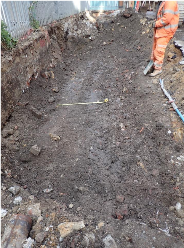
Figure 1: Overview of Trench, facing west
