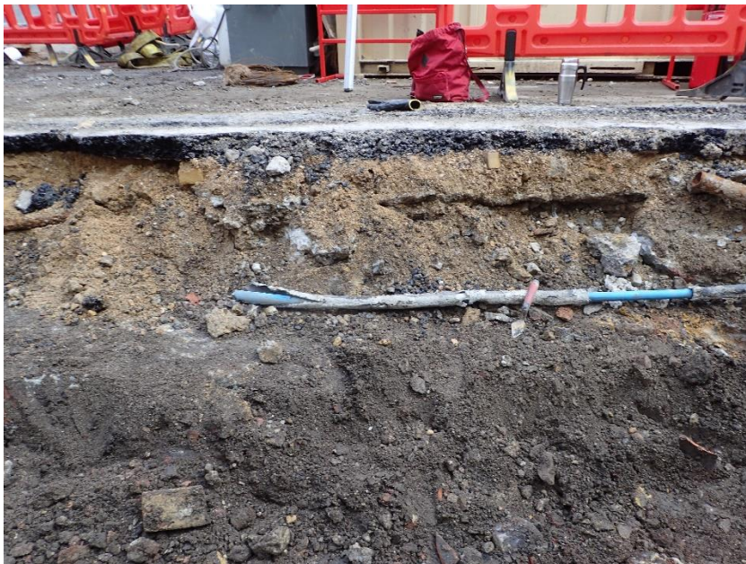
Figure 2: Section of Trench, facing north
