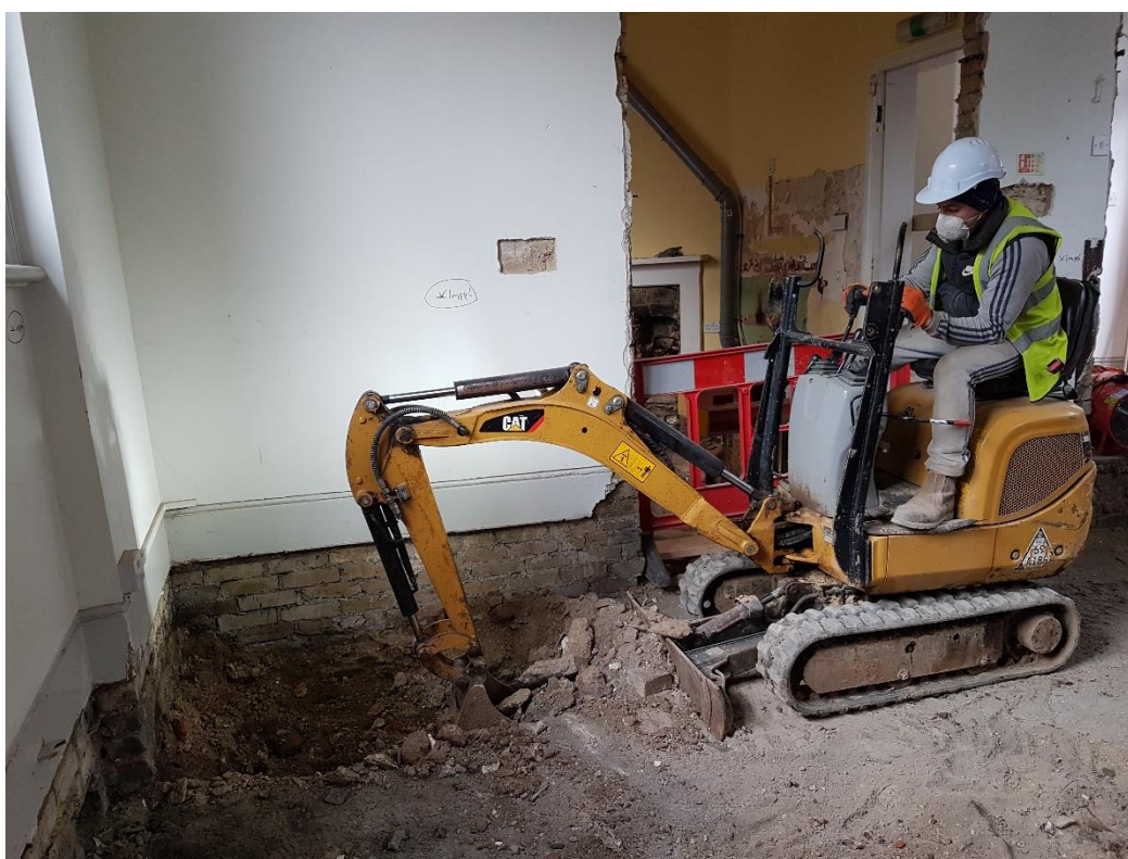
Plate 2: Excavation in progress, Trench 4, looking south.
