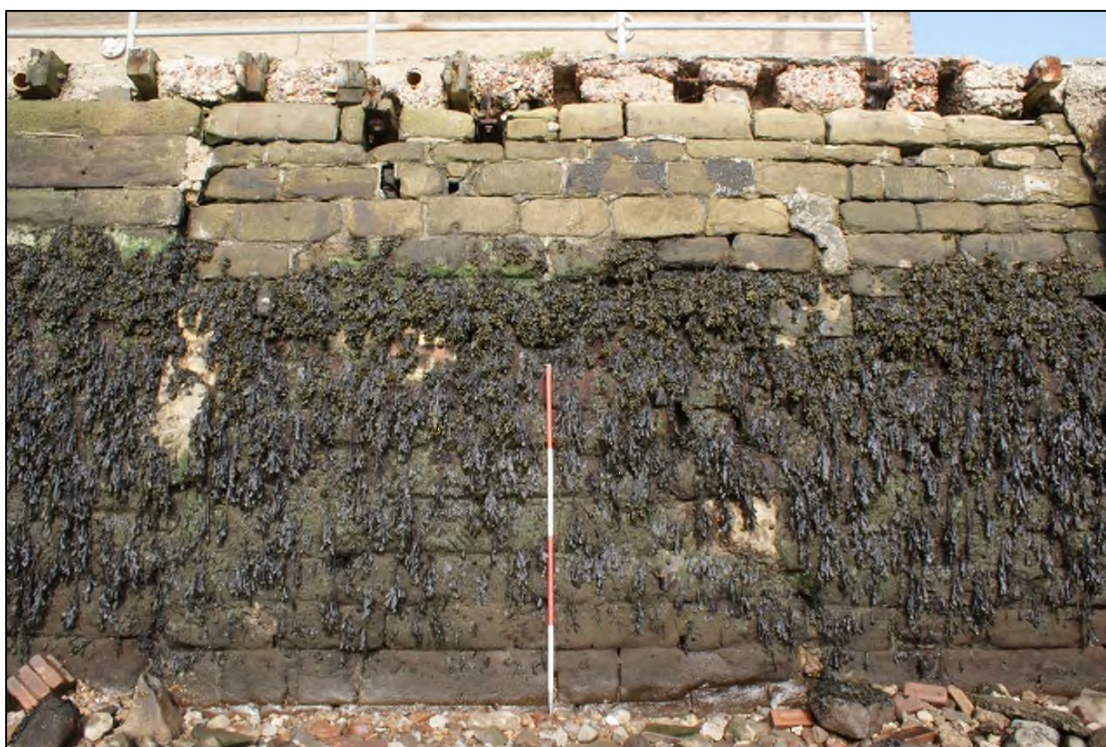
Plate 4: ESE facing elevation of NNE-SSW aligned quayside wall showing concrete and timber deck, View WNW, 2m scale.
