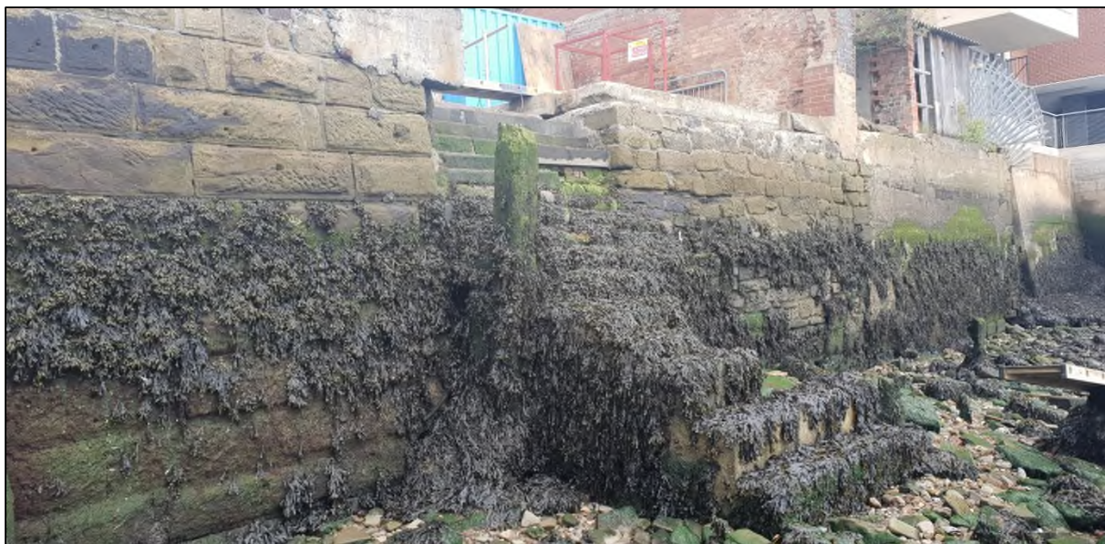
Plate 15: Staircase leading to foreshore, View NNW.
