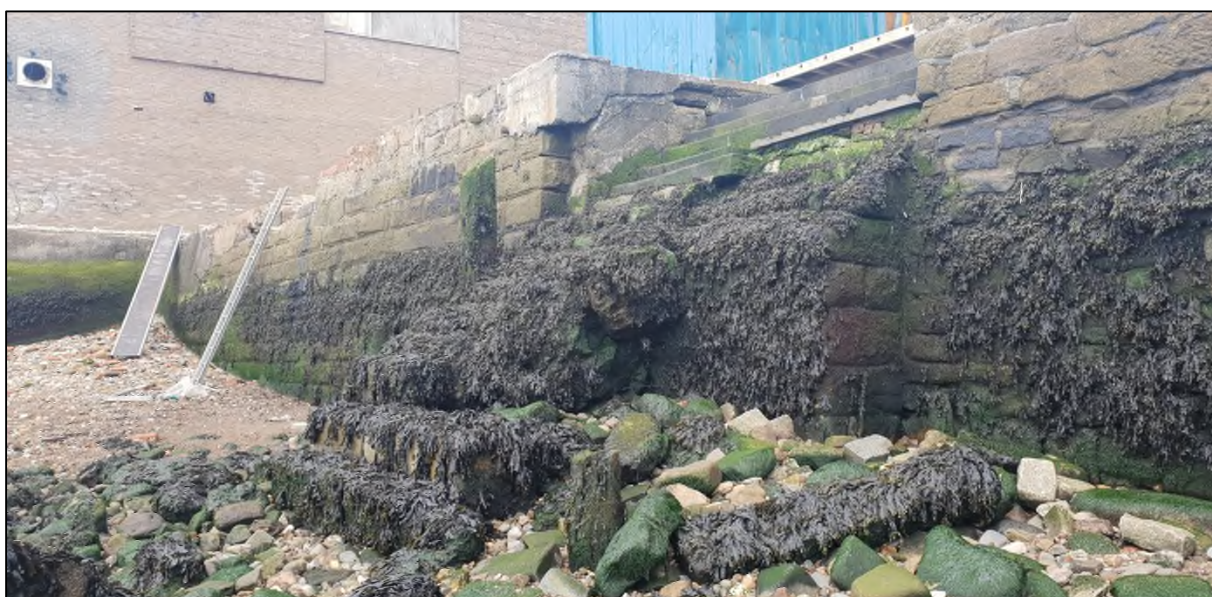
Plate 16: Staircase leading to foreshore, View SW.
