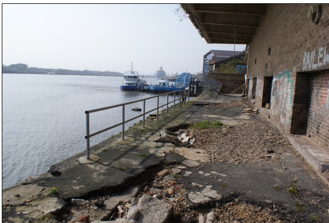
Plate 12: General view from top of NNE-SSW aligned quayside wall, View north.
