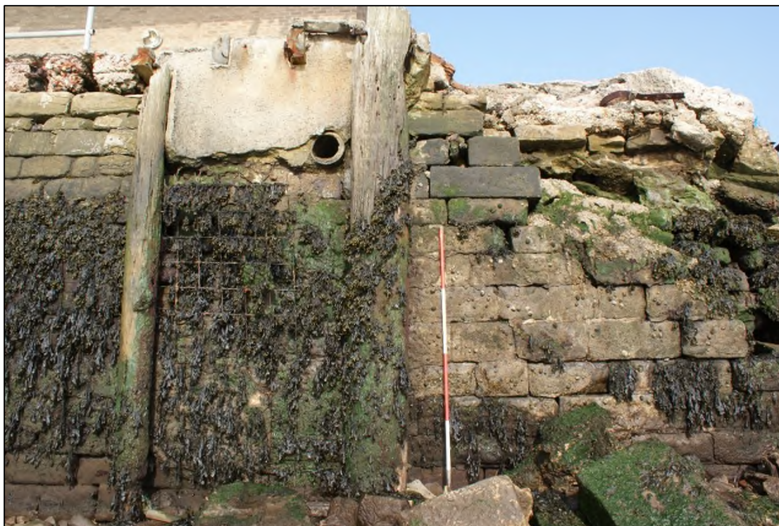
Plate 3: ESE facing elevation of NNE-SSW aligned quayside wall showing timber mooring posts and drain, View WNW, 2m scale.
