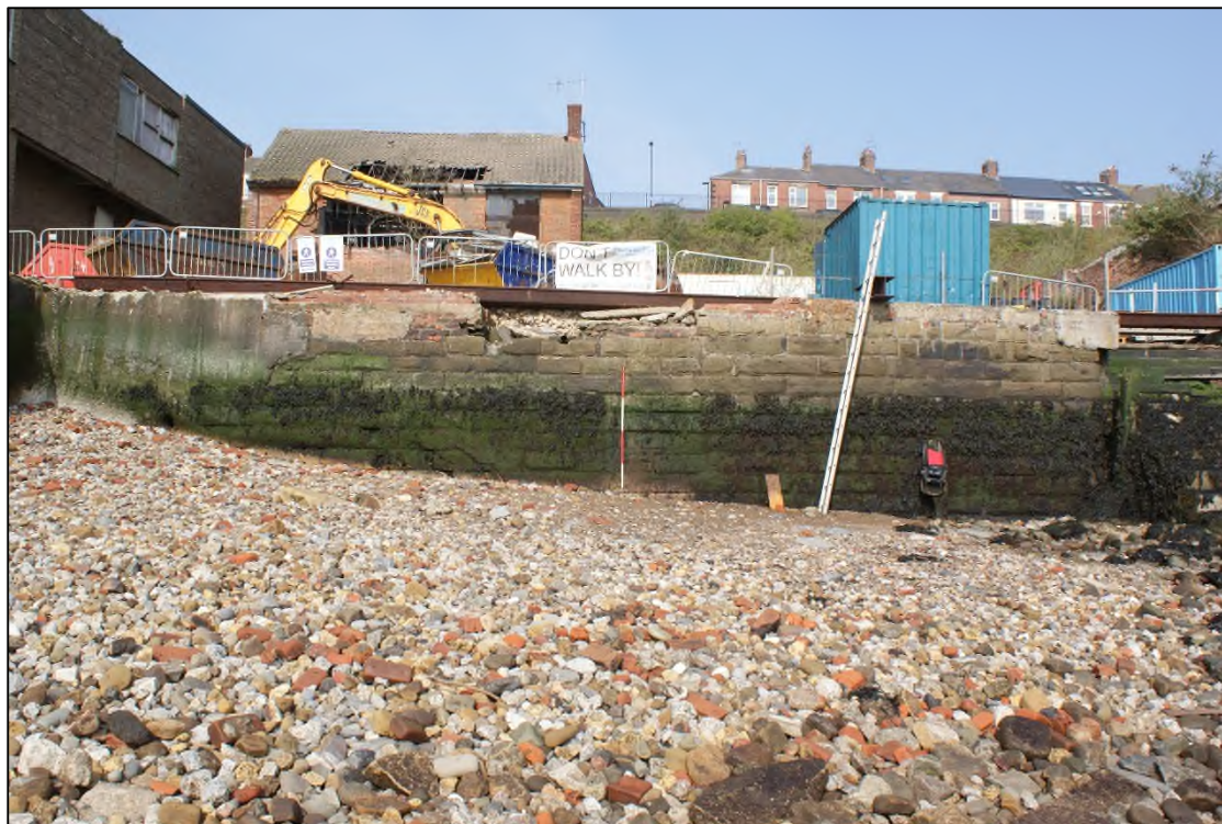
Plate 13: NNE-SSW aligned quayside wall facing property 30, View ENE, 2m scale.
