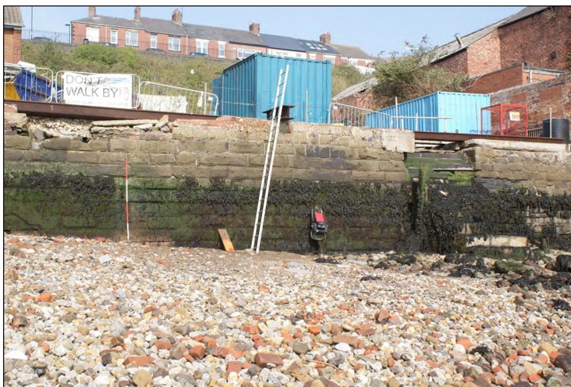
Plate 14: NNE-SSW aligned quayside wall facing property 30, View ENE, 2m scale.
