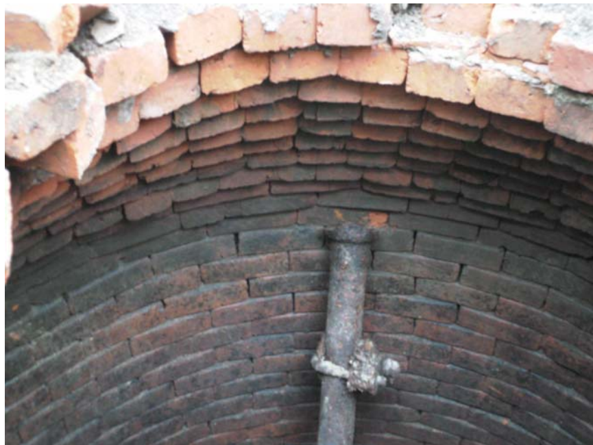
Plate 2. Structure [8]. Detail showing iron pipe, brick lining and dome.
