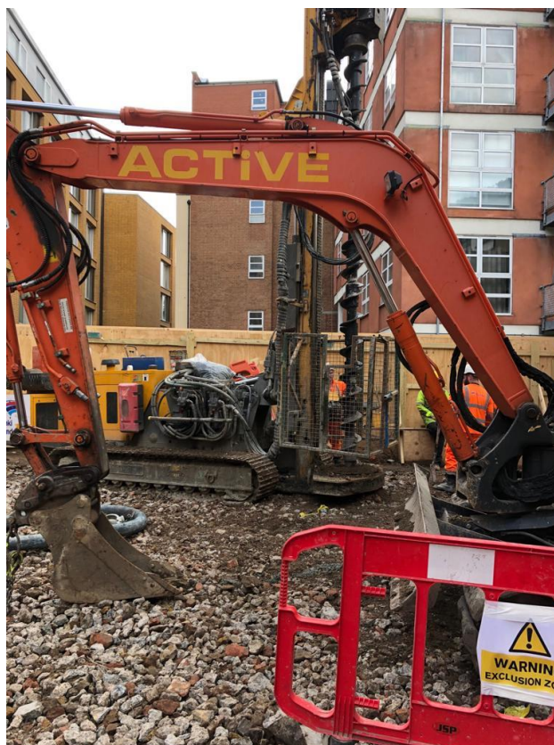
Plate 8: Piling works in progress, looking east
