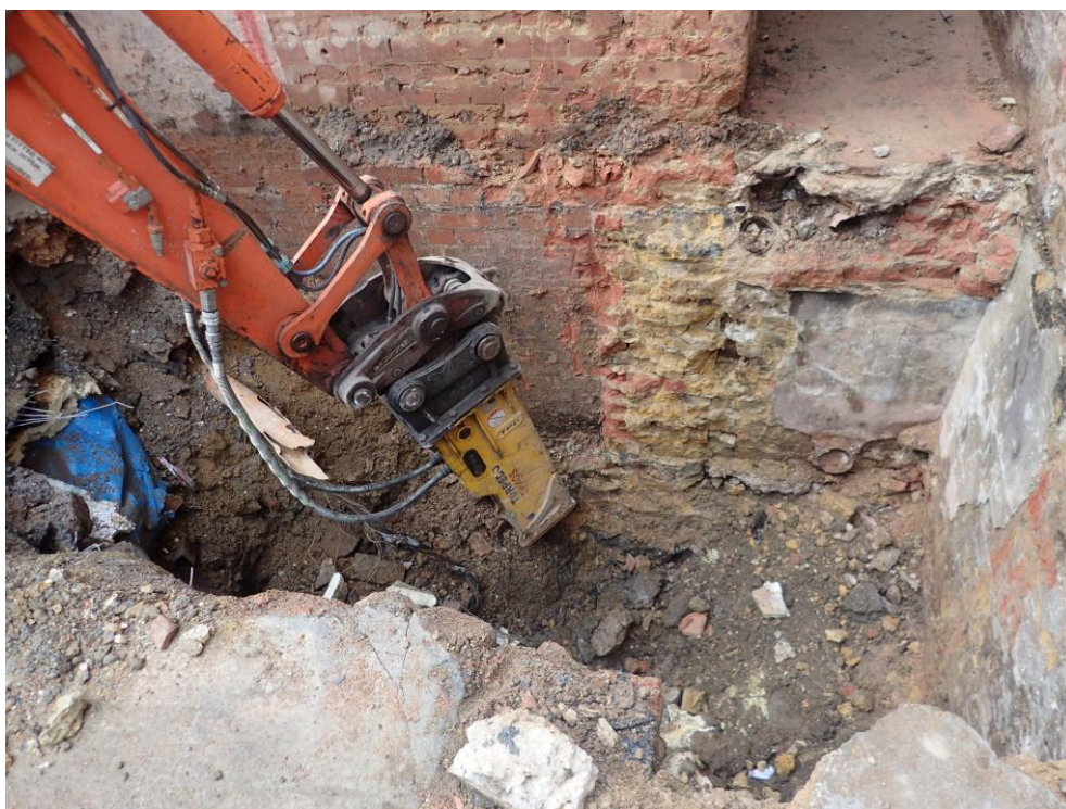
Plate 6: Trench 2 under excavation, looking west
