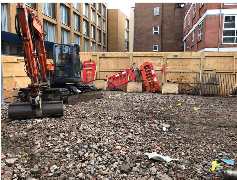
Plate 7: The site prepared for piling works, looking east-south-east
