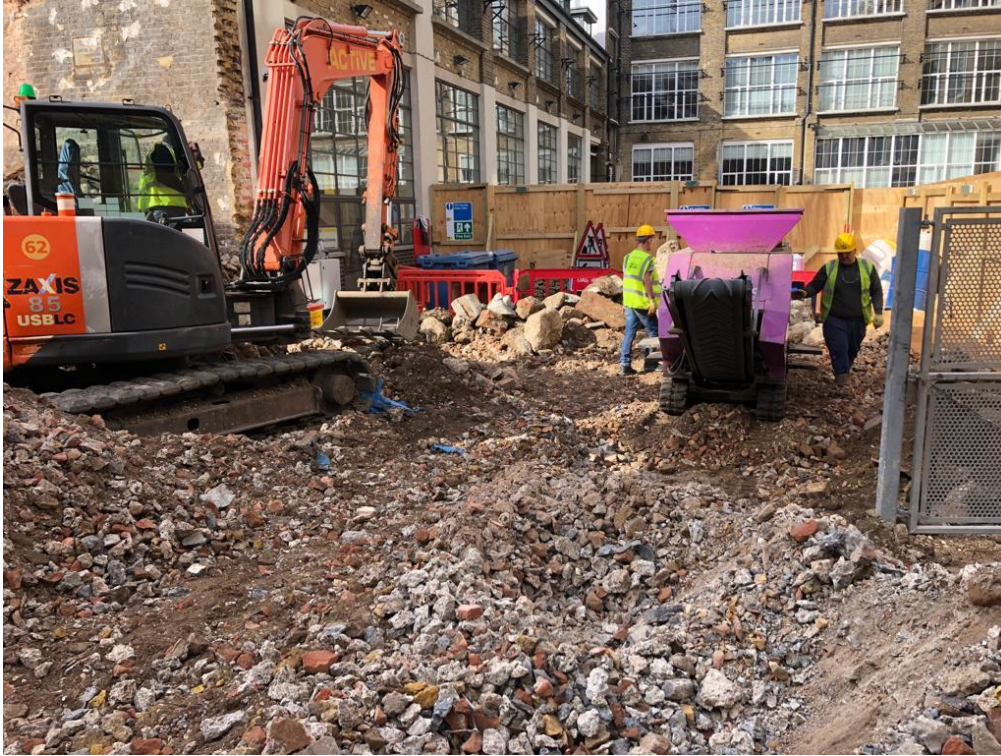
Plate 2: General view of the site during demolition, looking west
