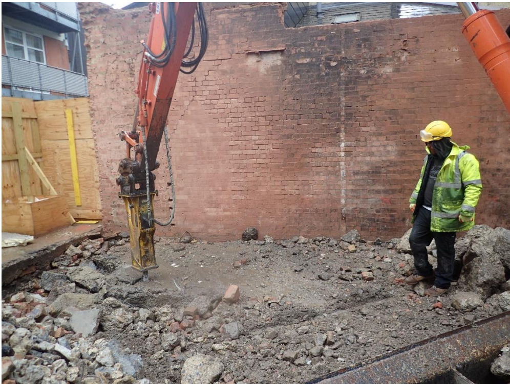
Plate 1: Breaking up of the concrete slab, looking south-south-west
