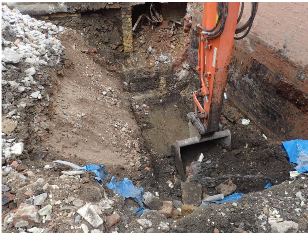
Plate 5: Trench 1, looking south-east
