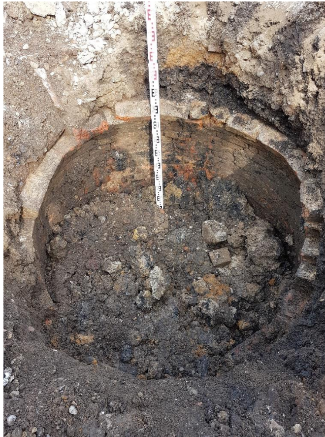
Plate 5: Soakaway [4], looking north-west
