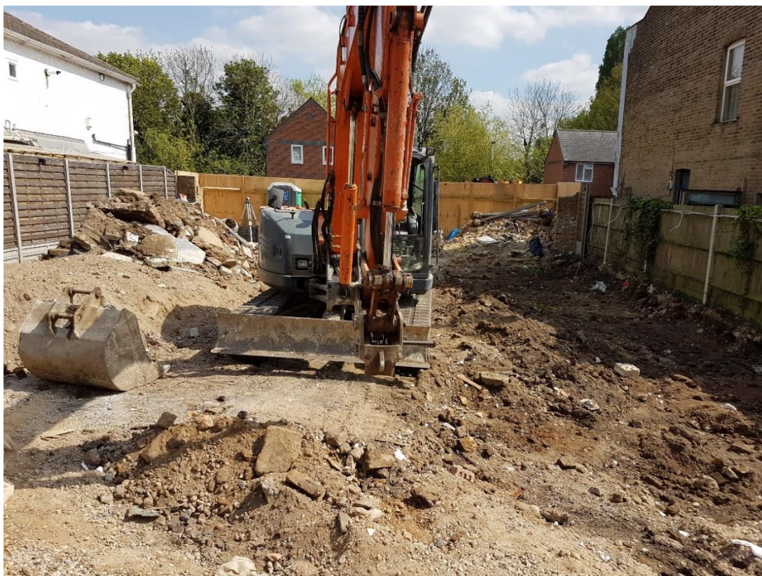
Plate 1: Surface removal and ground reduction, looking north-west.
