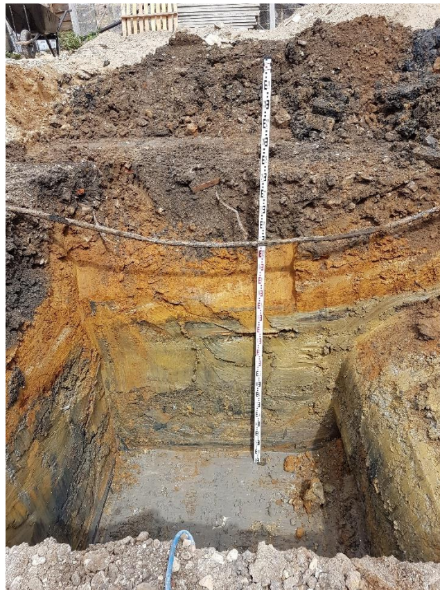
Plate 6: Pit after removal of the soakaway [4], looking north-west
