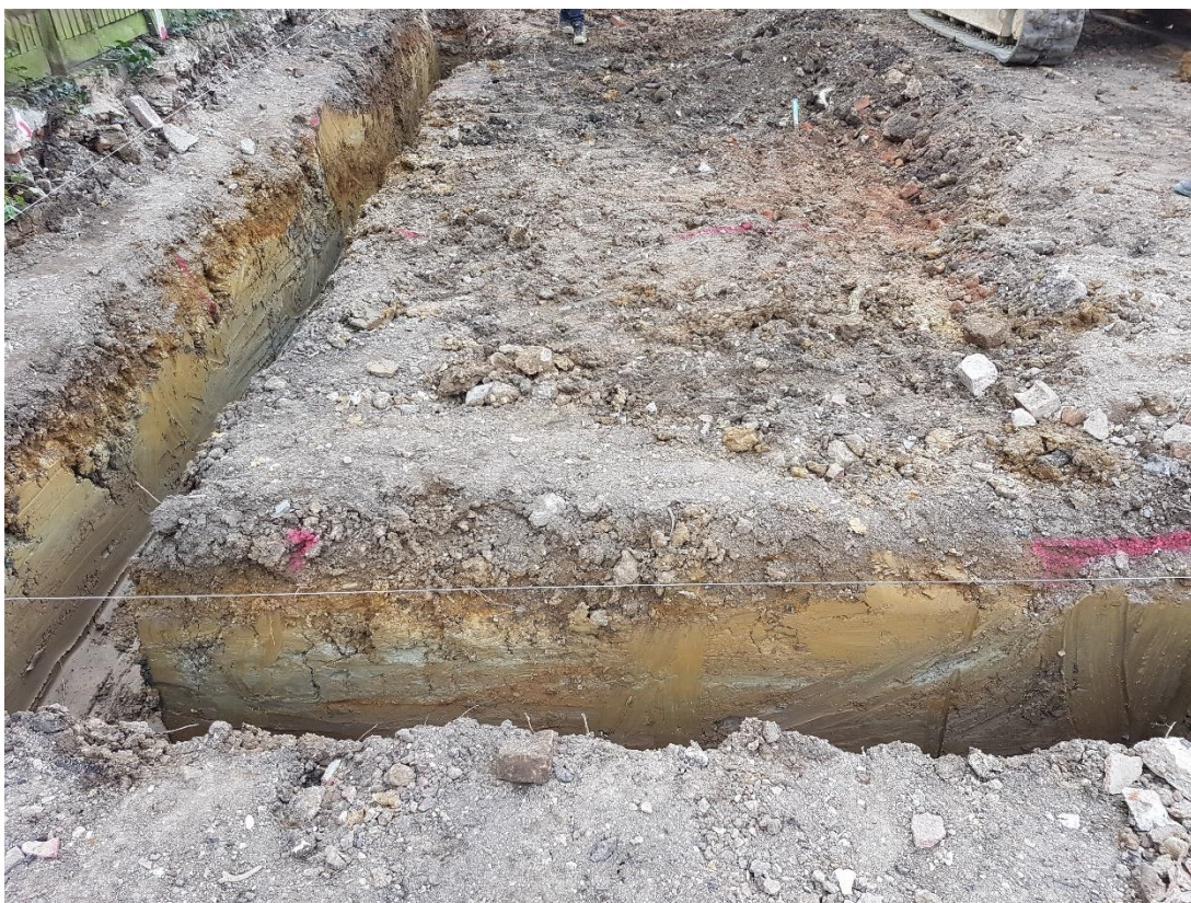
Plate 2: Trench 1, looking north-west
