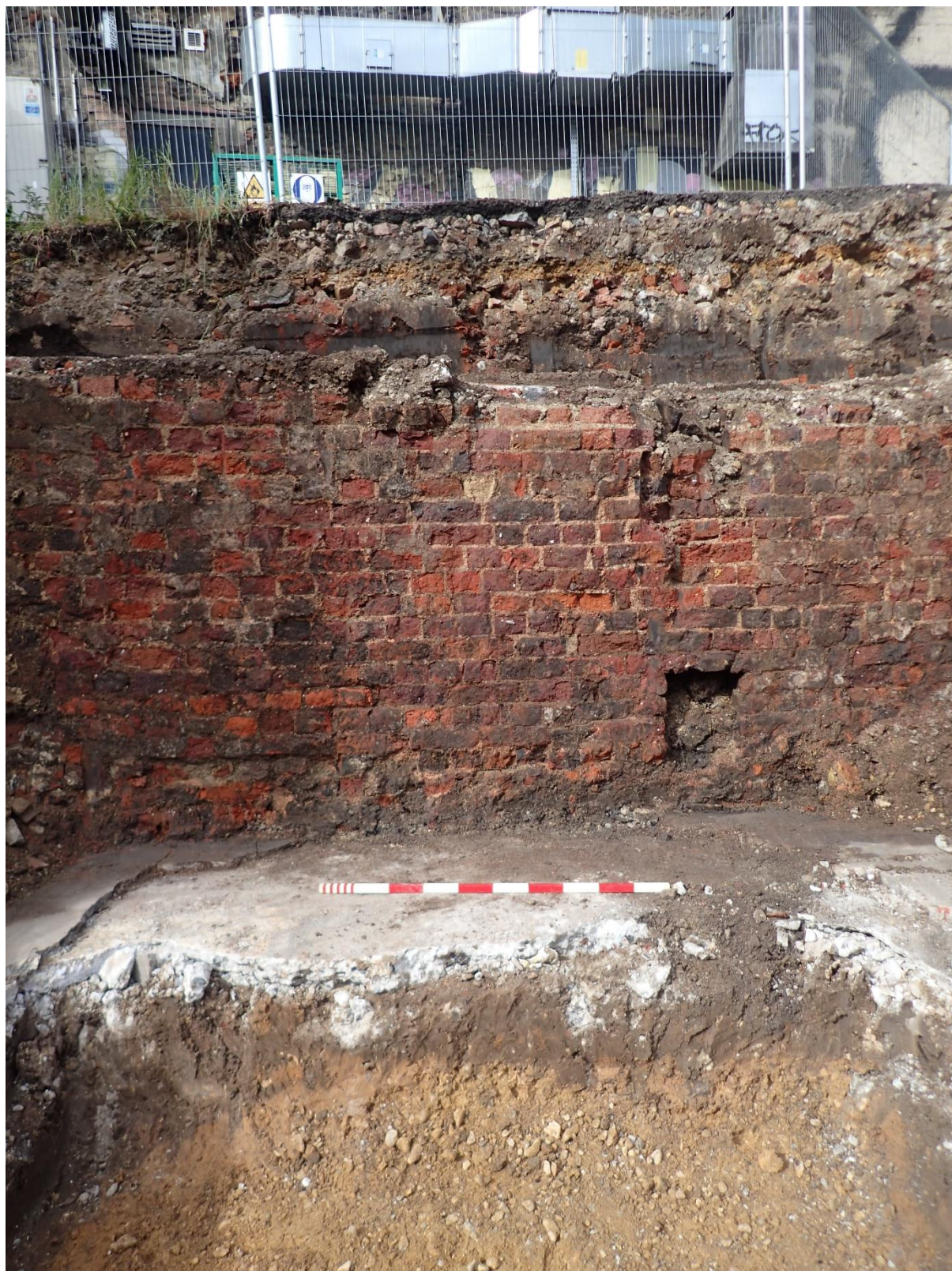
Plate 2: West facing view of basement structure [101]/[103] (1m scale)
