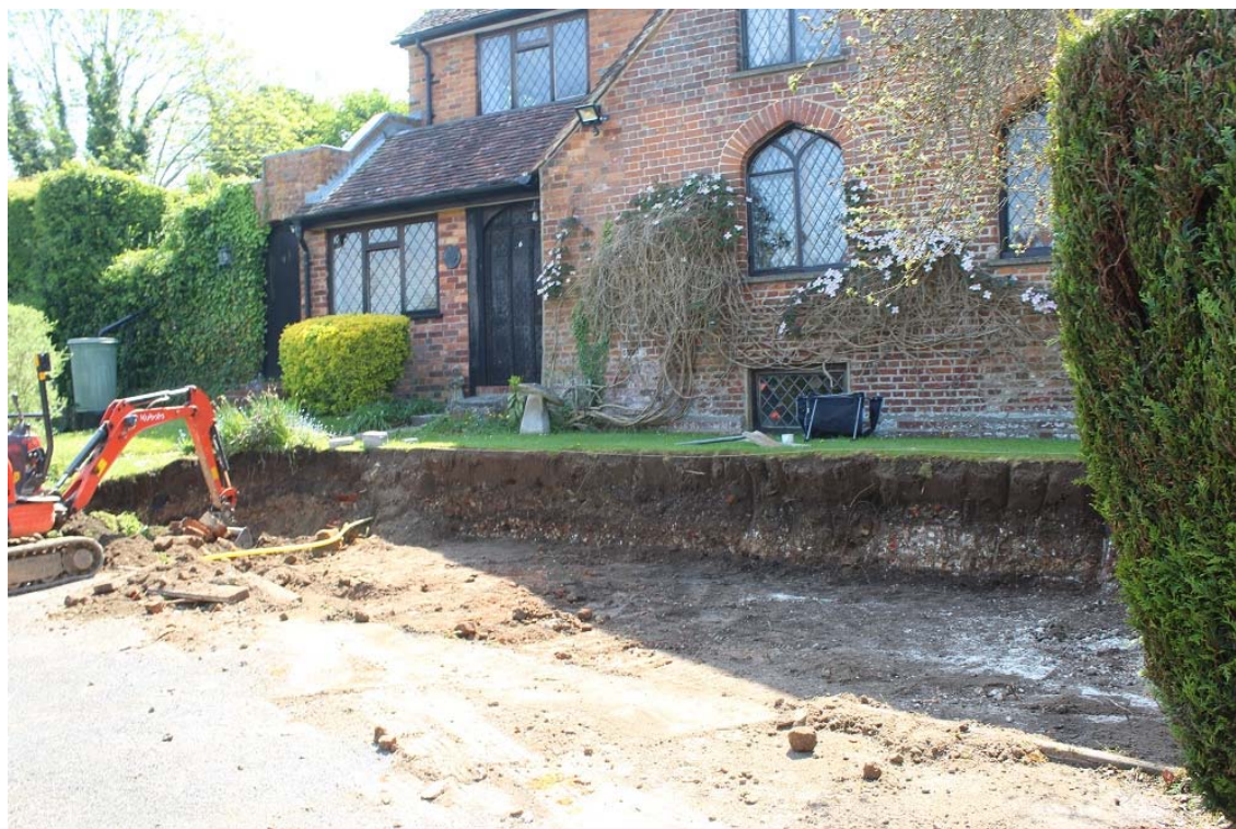
Plate 3. Image of main Site section and stripped area. View south-east.
