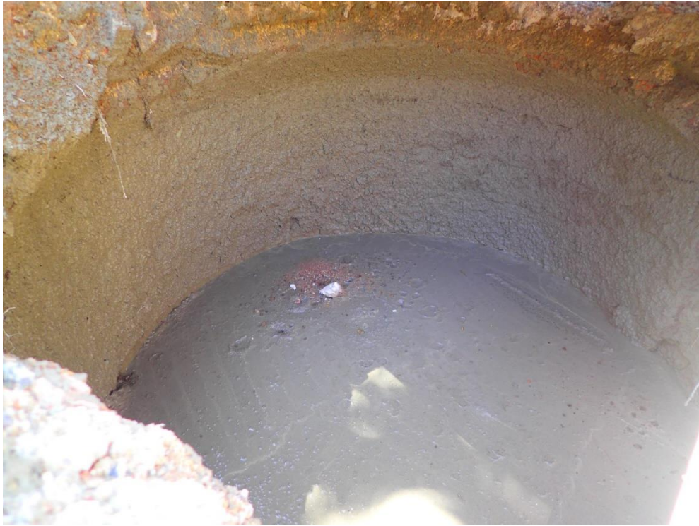
Plate 2, view to south-west, no scale but c.2m in diameter: brick-built cistern [11]
