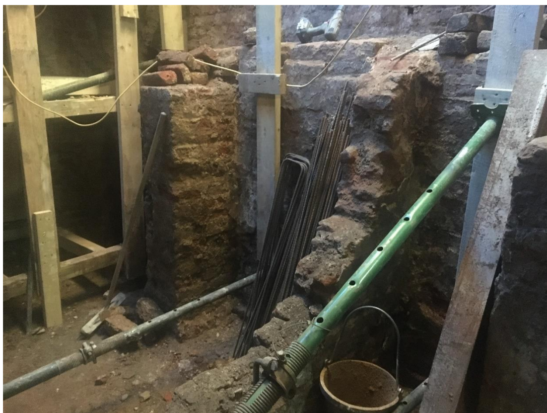
Plate 2: Wall [100] and partitions, looking north-west
