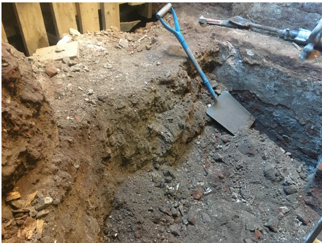
Plate 1: Basement backfill [101], looking north
