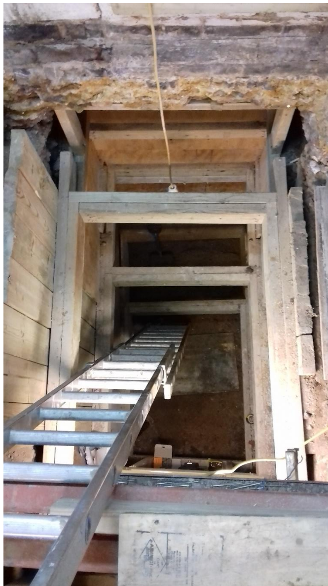
Plate 4: One of the excavated pits within the basement.
