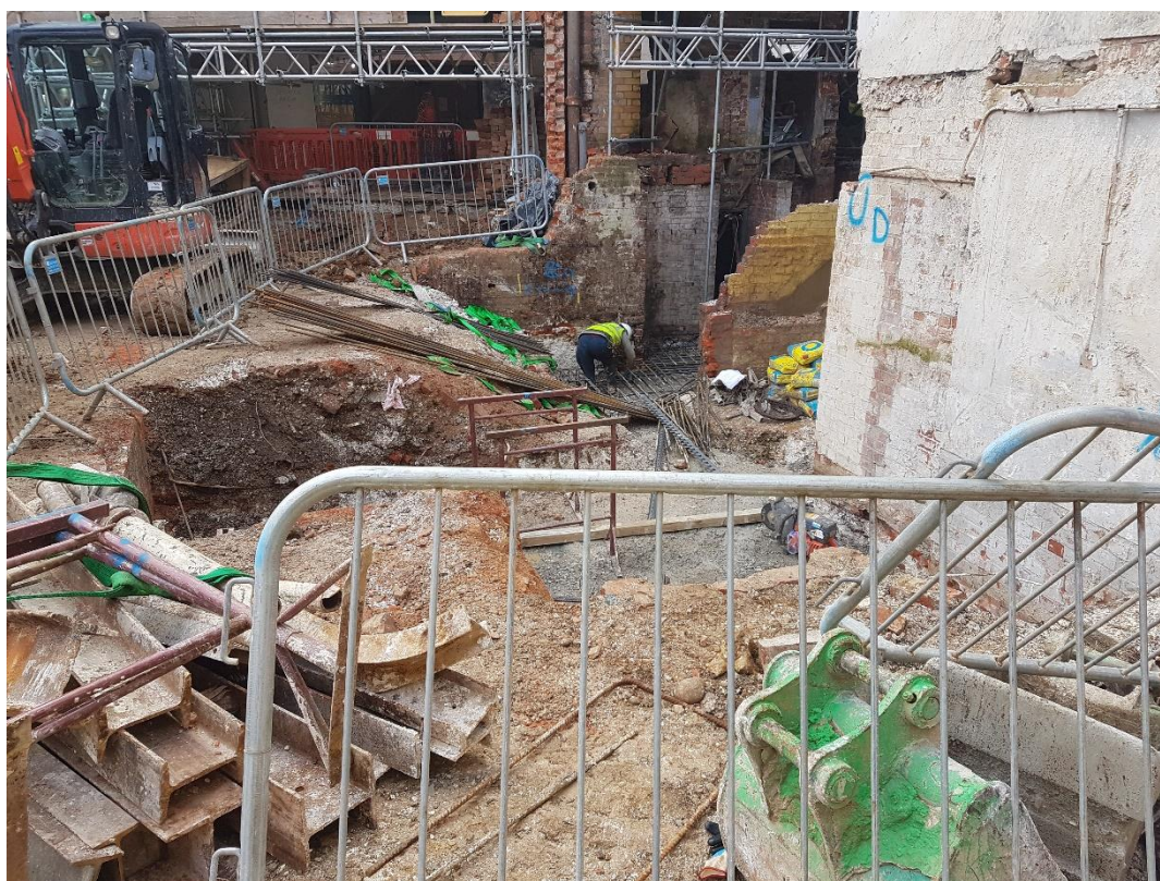
Plate 4 View to the south-west of basement excavations
