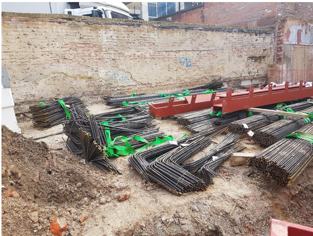
Plate 7 View to the south-east
