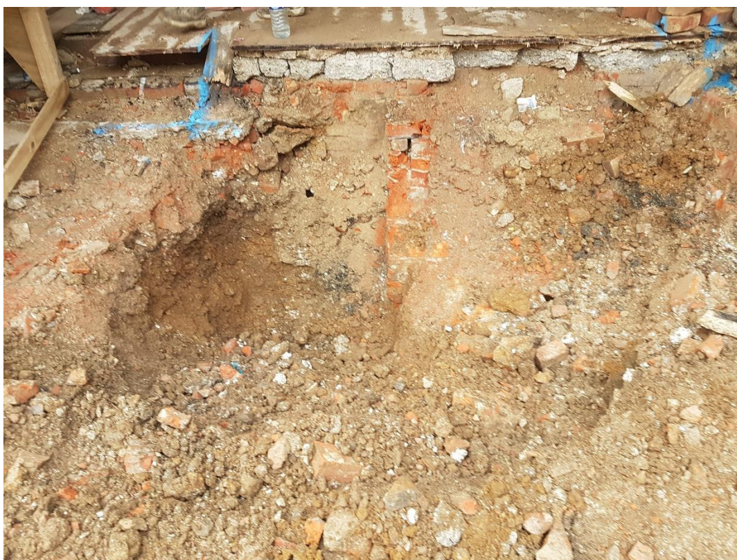
Plate 8 View to the south of grubbed out area
