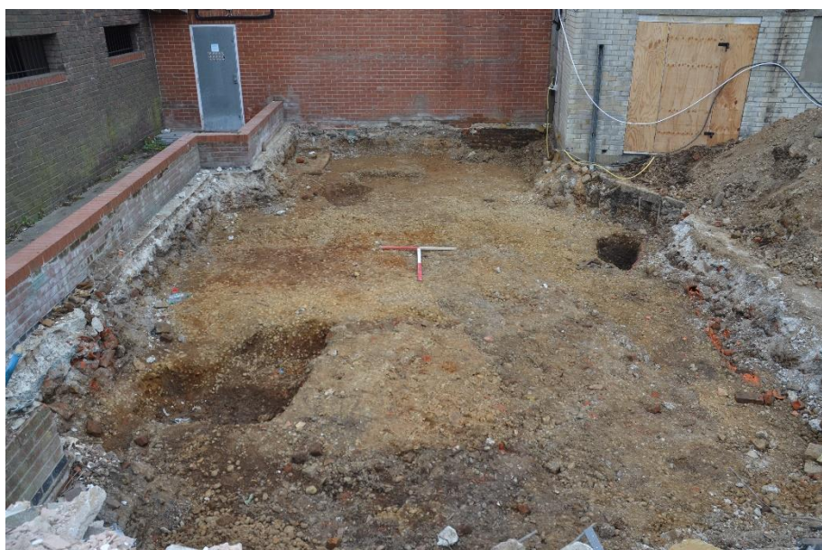
Plate 2: View west of the site (excavation)
