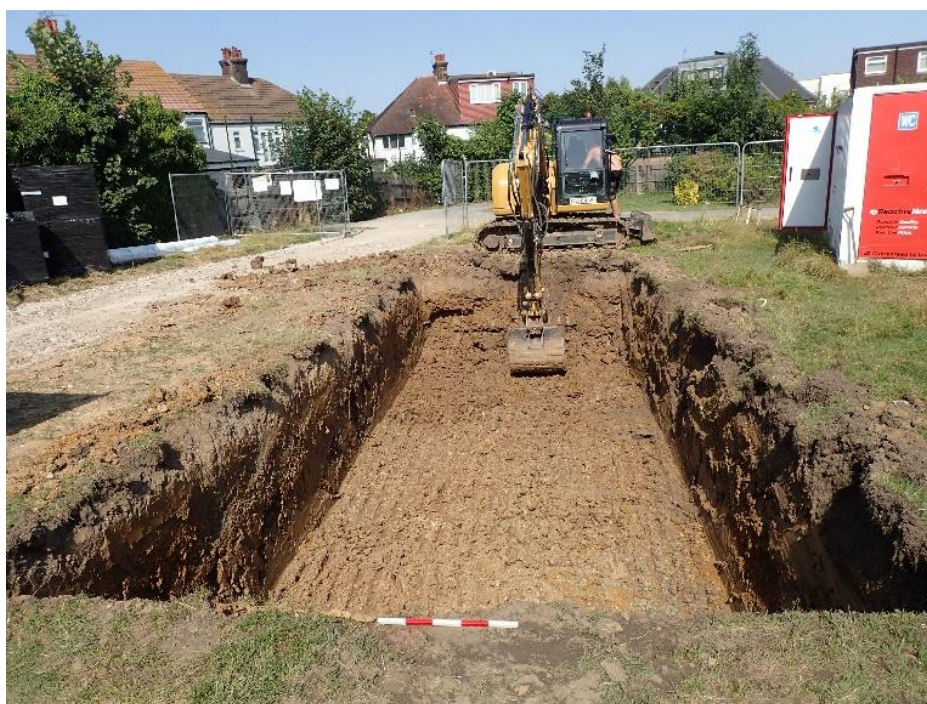
Plate 3: Boiler Trench, view to the west, scale 0.5m
