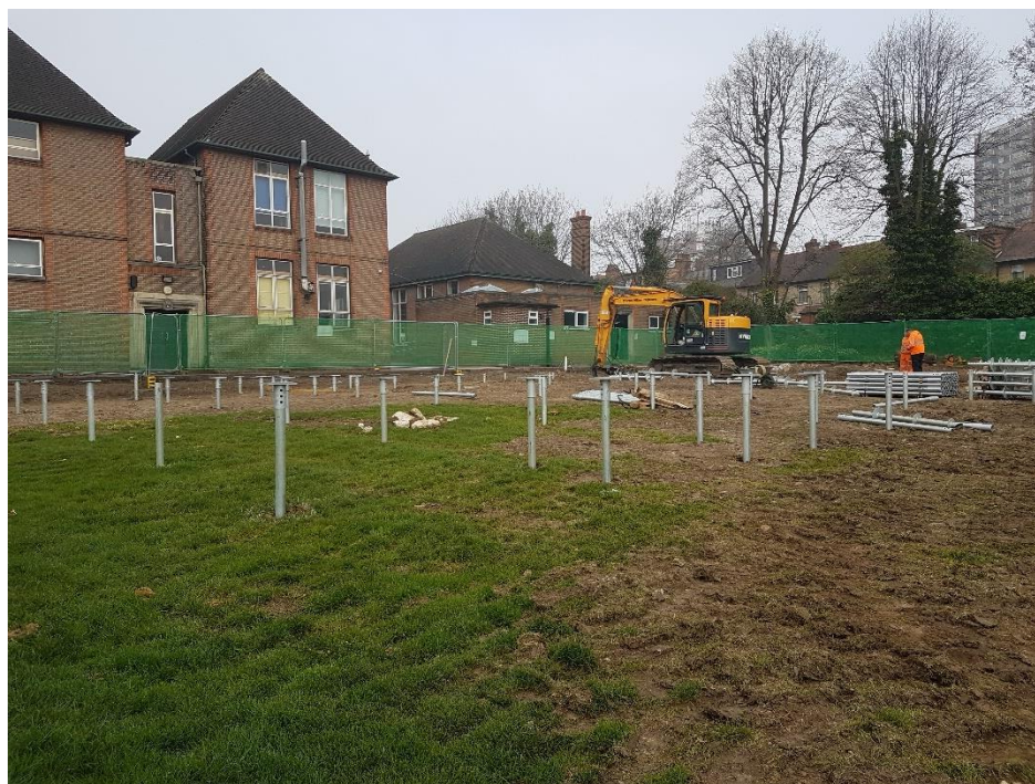
Plate 6: Inserted screw piles, view to the north-west
