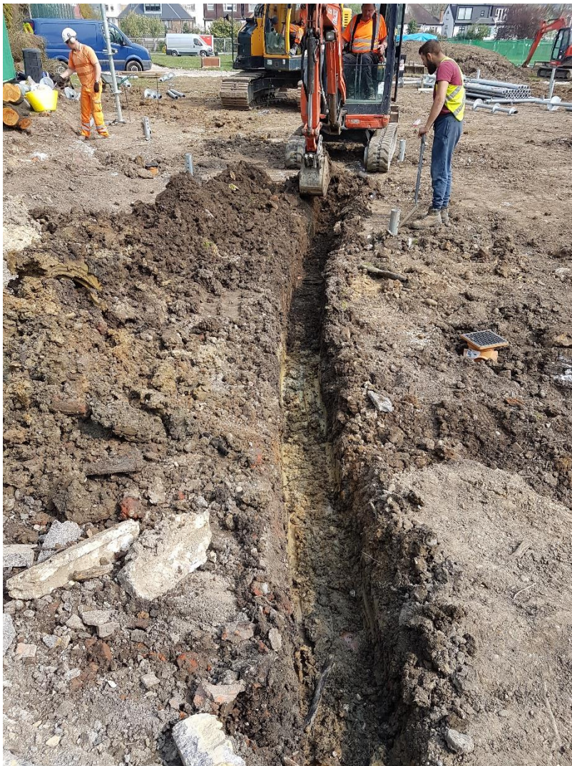
Plate 1: Excavation of a drainage trench, view to the south
