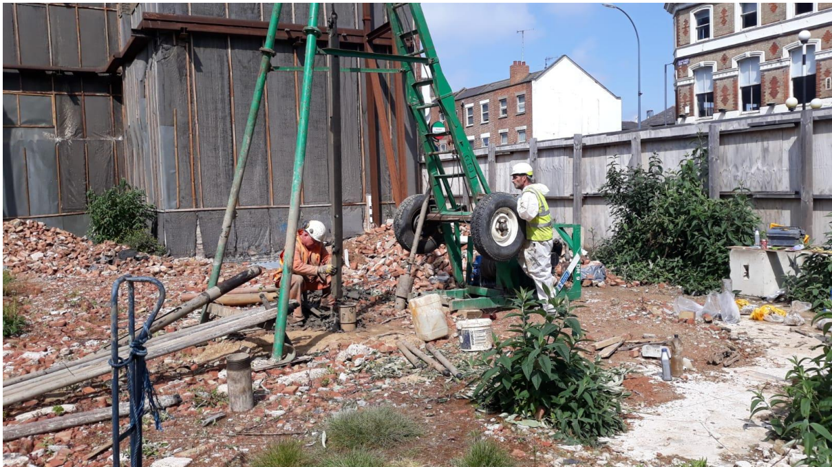
Plate 3: Borehole 101 during the works, looking north-west.
