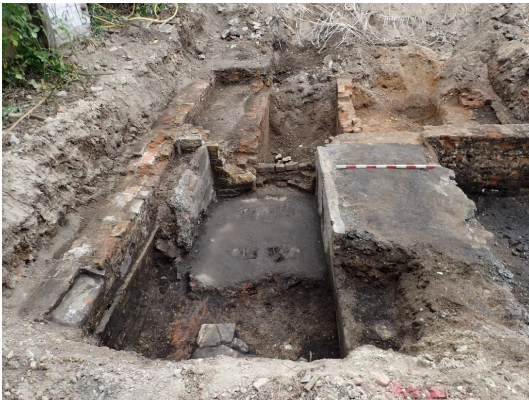
Plate 6: Trench 2, looking south, north-south brick walls [3], [2] and [1] (from left to right), cast concrete walls [8] and [10] and floors [7] and [9] in the foreground.
